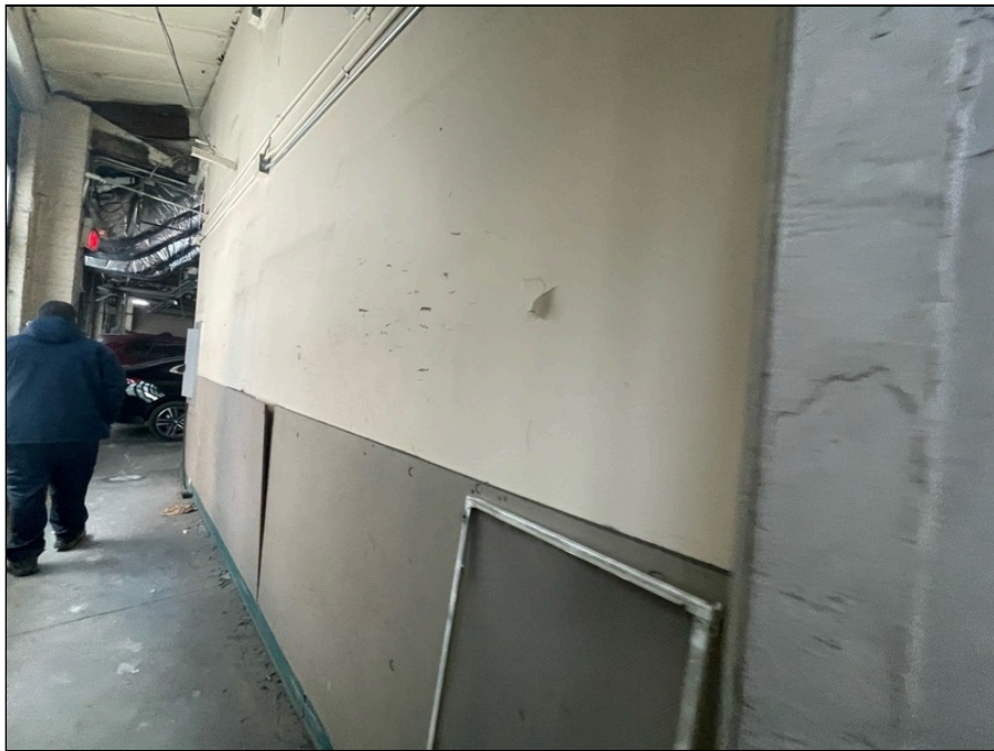
Photo 78: Second floor finishes
