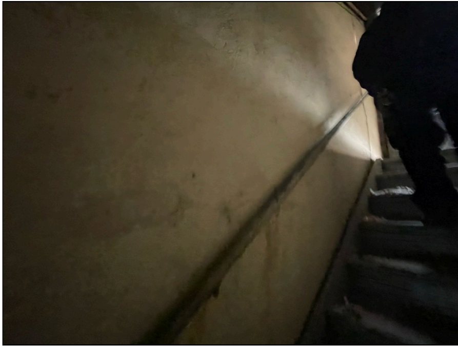
Photo 177: Stairwell to the roof
