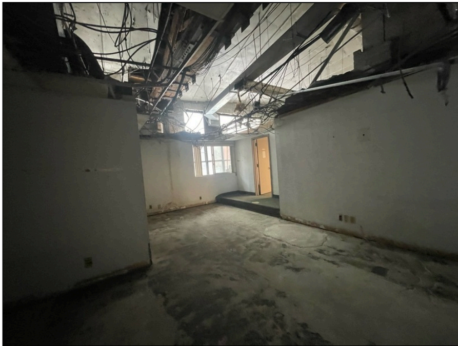
Photo 146: Second floor finishes
