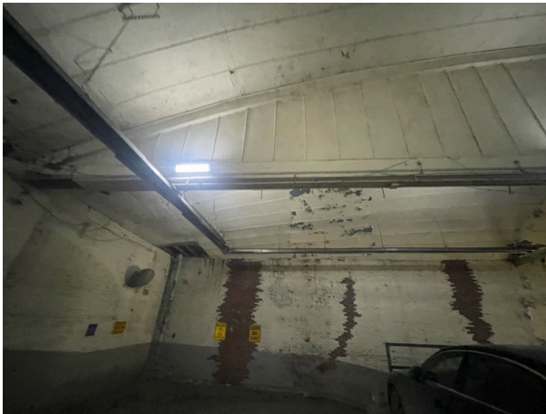
Second floor finishes
