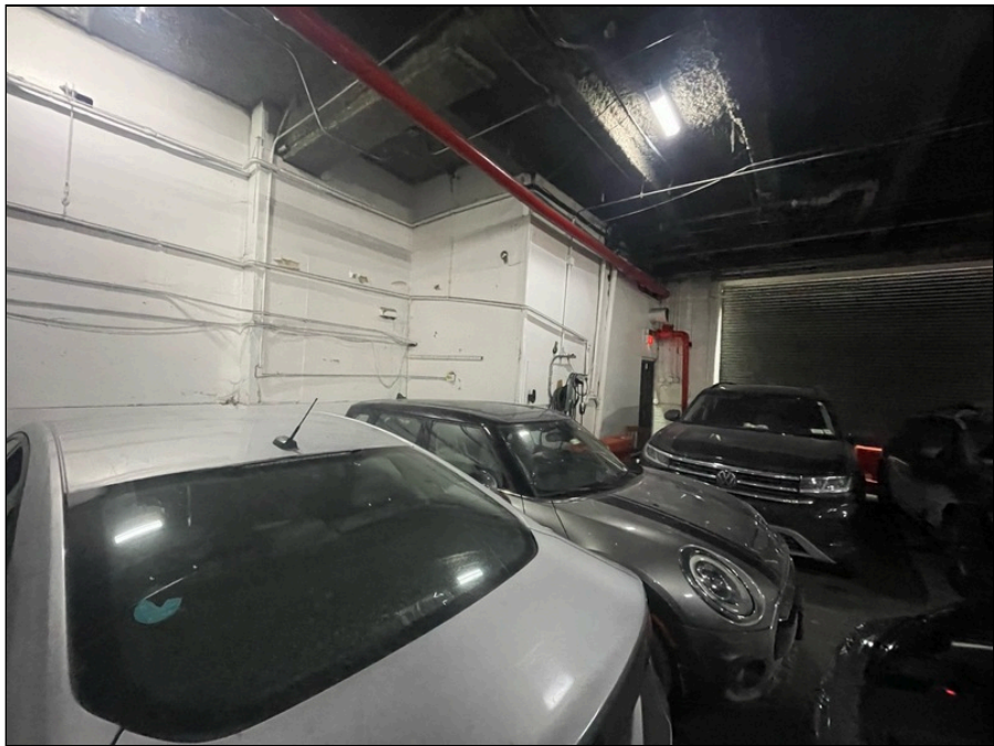
Photo 33: First floor parking garage finishes
