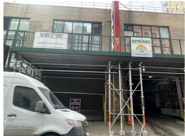
North side of the building
