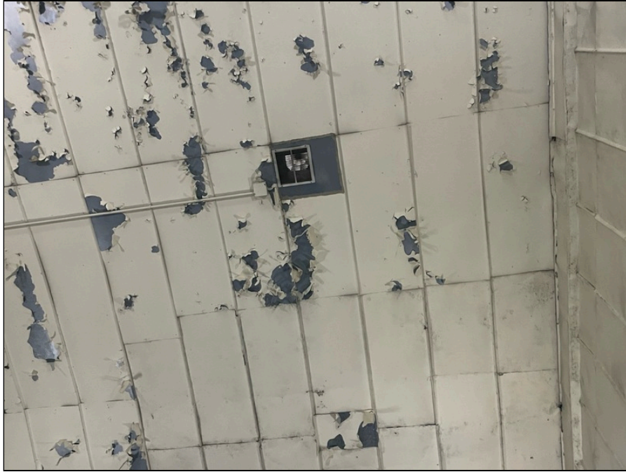
Photo 203: Second floor finishes
