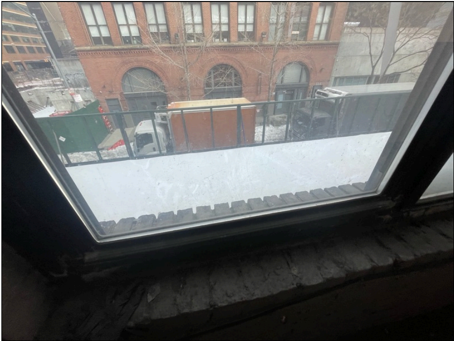
Photo 80: Second floor finishes
