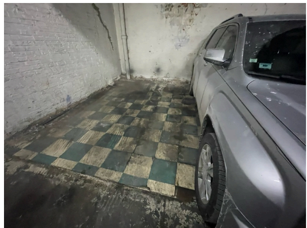
First floor parking garage finishes
