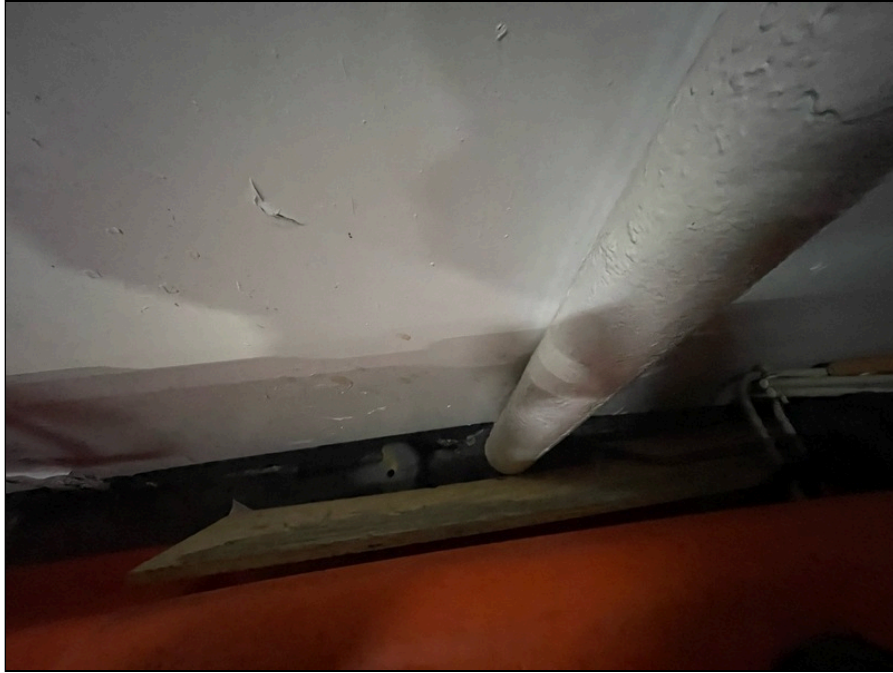
Photo 35: First floor parking garage finishes
