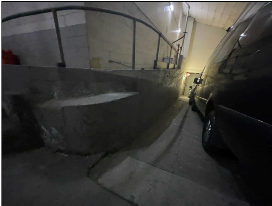
Photo 126: Second floor finishes
