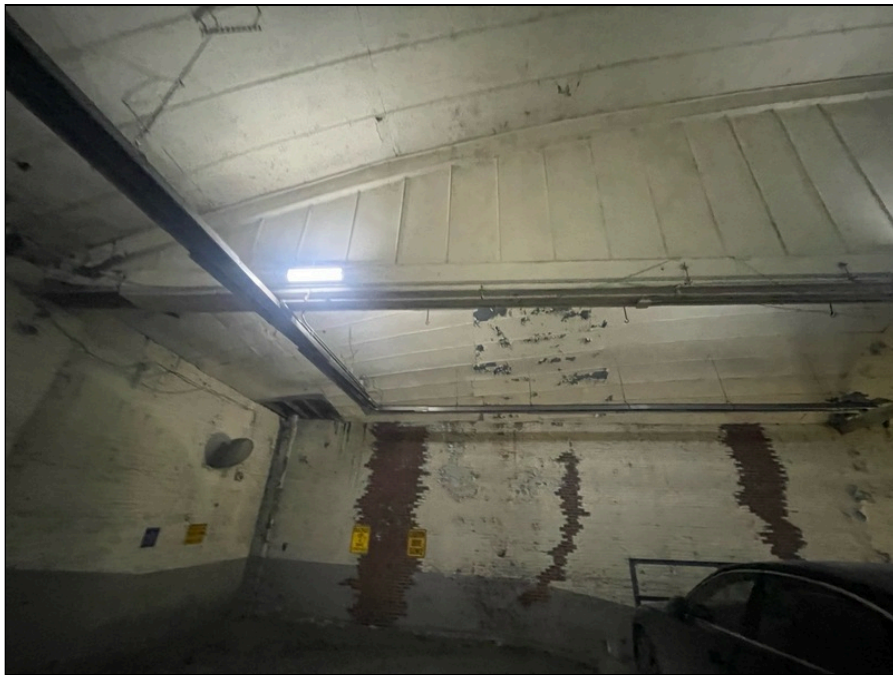
Photo 104: Second floor finishes
