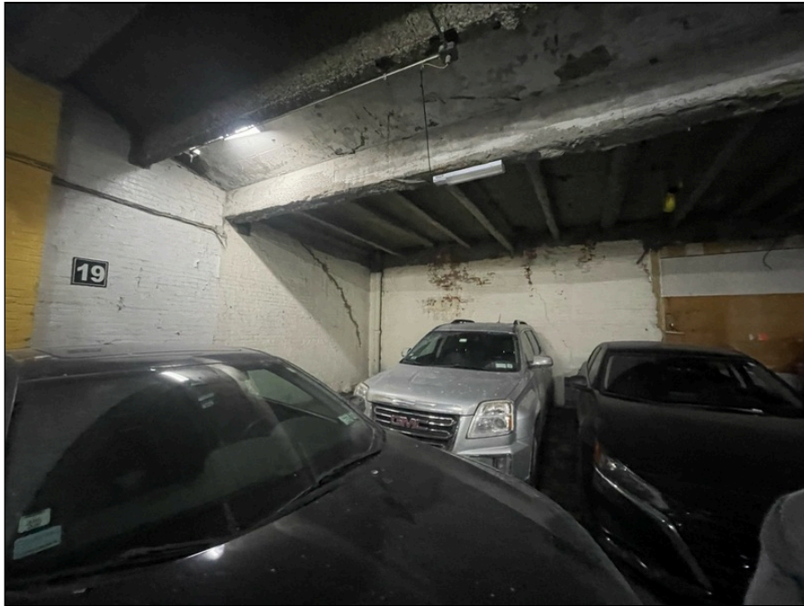
Photo 49: First floor parking garage finishes
