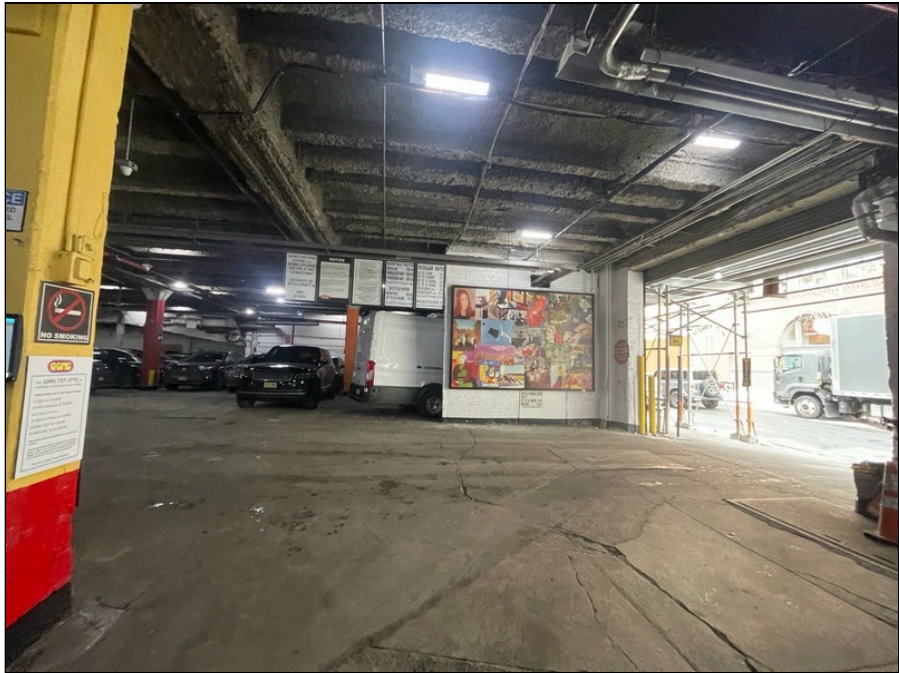
Photo 11: First floor parking garage finishes
