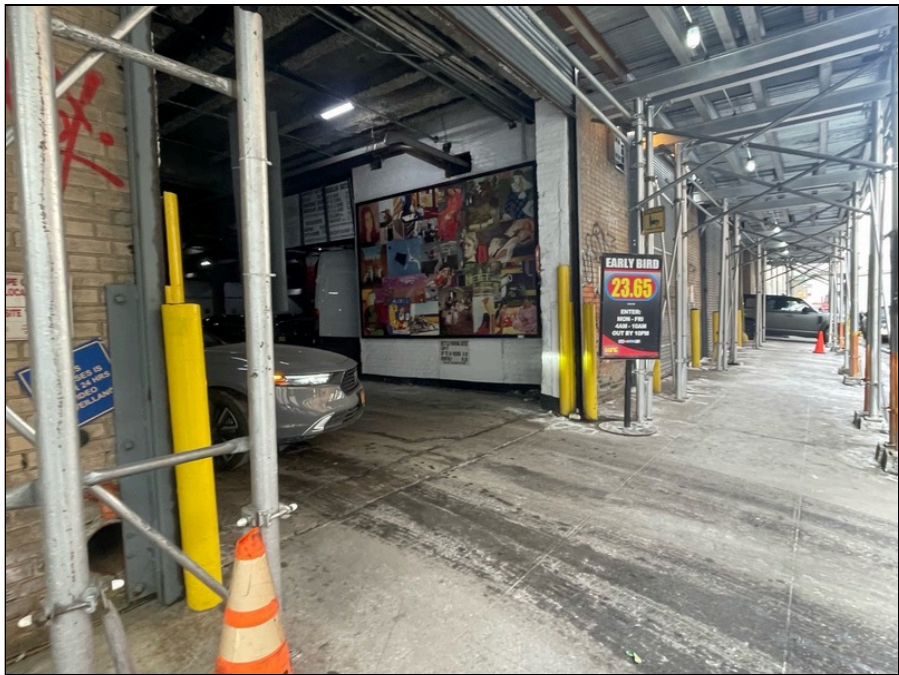
Photo 8: First floor parking garage finishes
