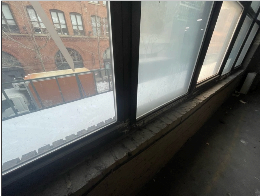
Photo 81: Second floor finishes
