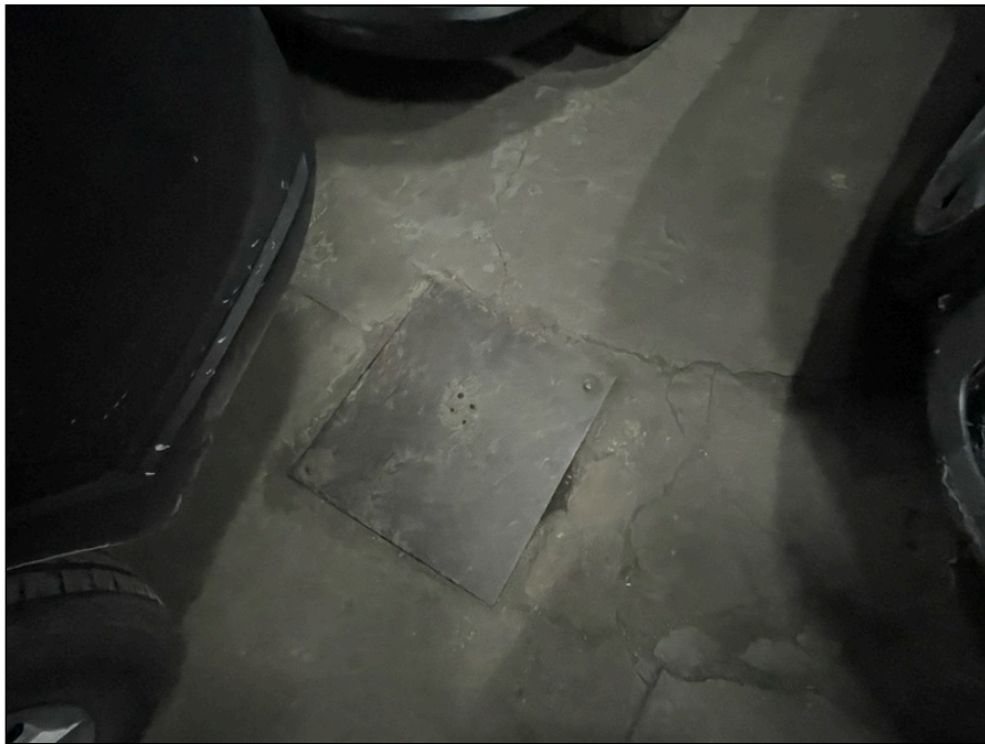
Photo 46: Floor drain, first floor
