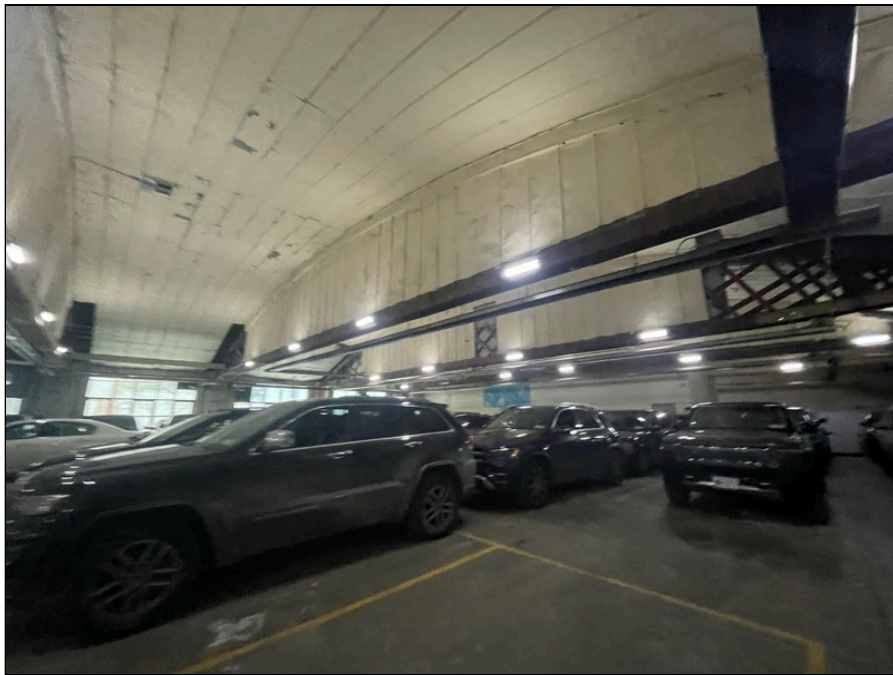
Photo 114: Second floor finishes
