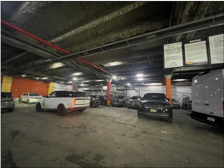
Photo 30: First floor parking garage finishes
