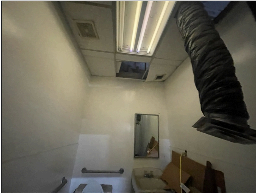
Photo 59: Bathroom finishes, first floor
