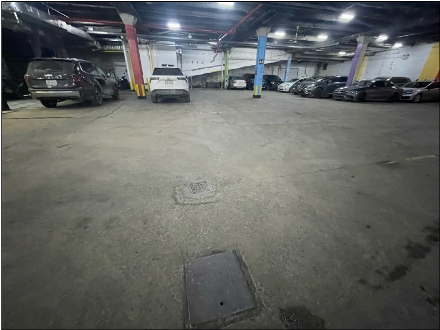
Photo 21: First floor parking garage finishes
