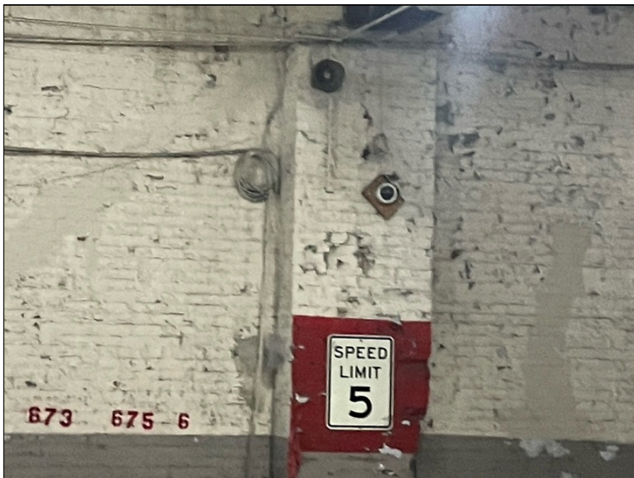
Photo 140: Second floor finishes
