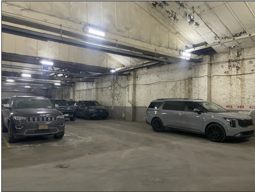
Photo 101: Second floor finishes
