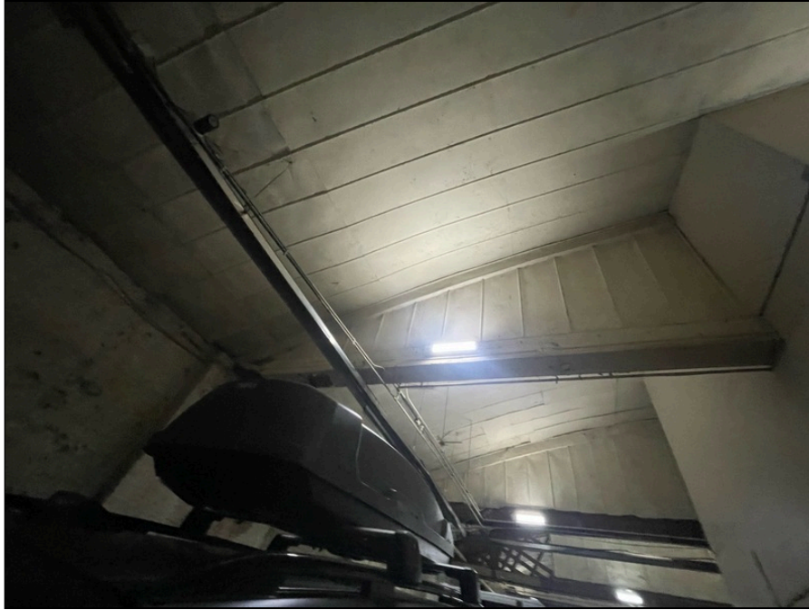
Photo 129: Second floor finishes
