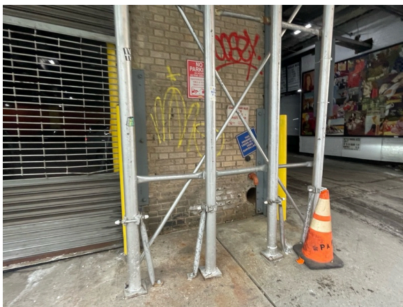
North side of the building
