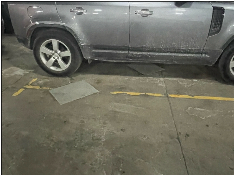
Photo 61: First floor parking garage finishes
