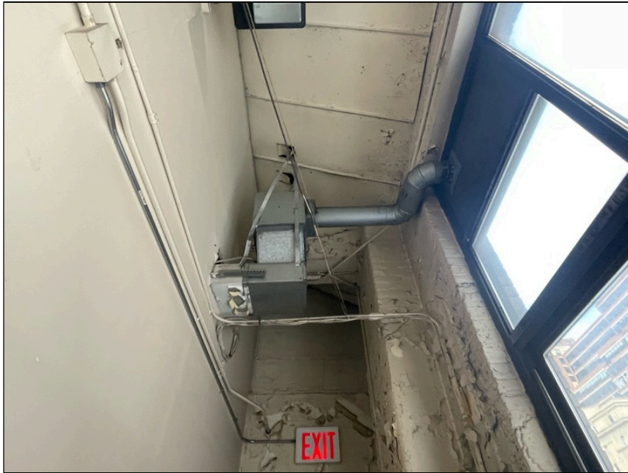
Photo 85: Second floor finishes
