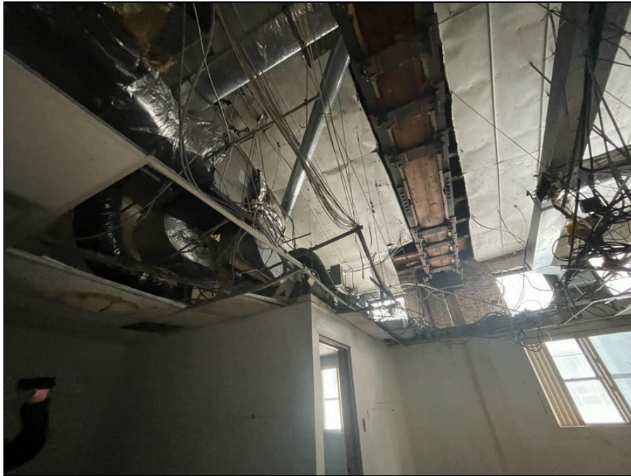
Photo 147: Second floor finishes
