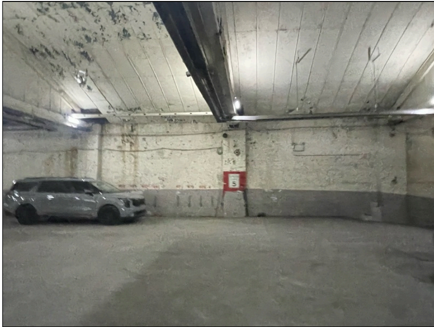
Photo 97: Second floor finishes
