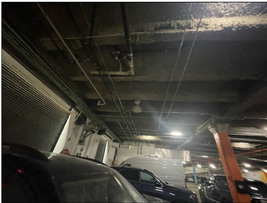
Photo 40: First floor parking garage finishes
