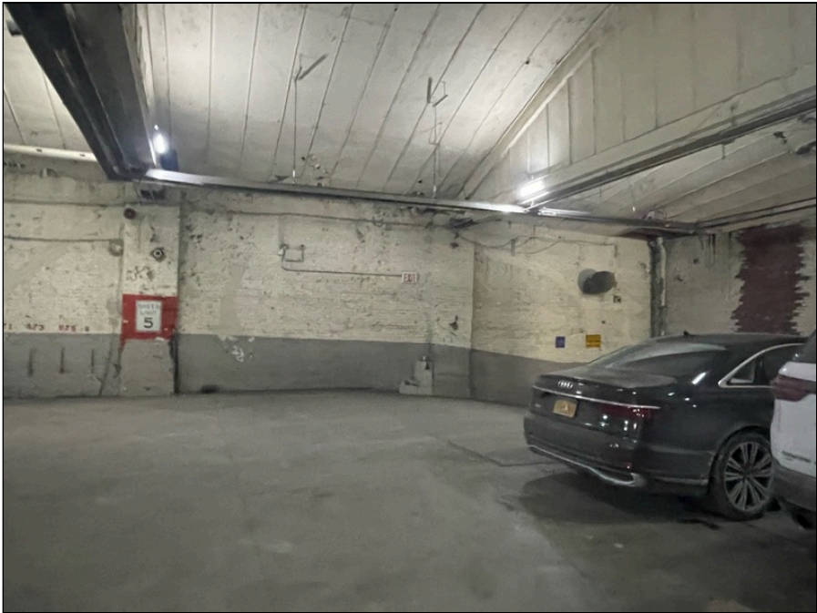
Photo 99: Second floor finishes
