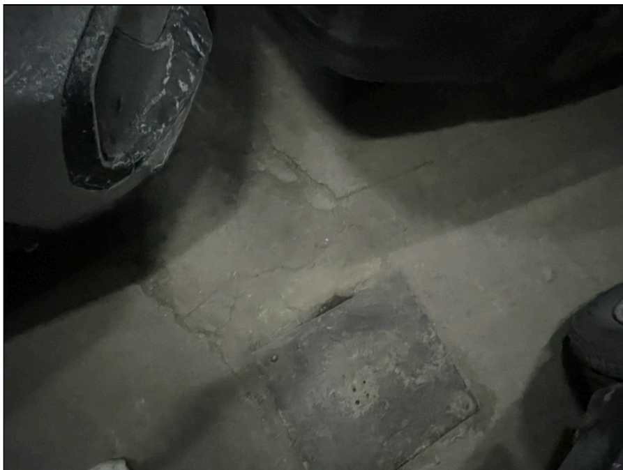
Photo 48: Floor drain, first floor
