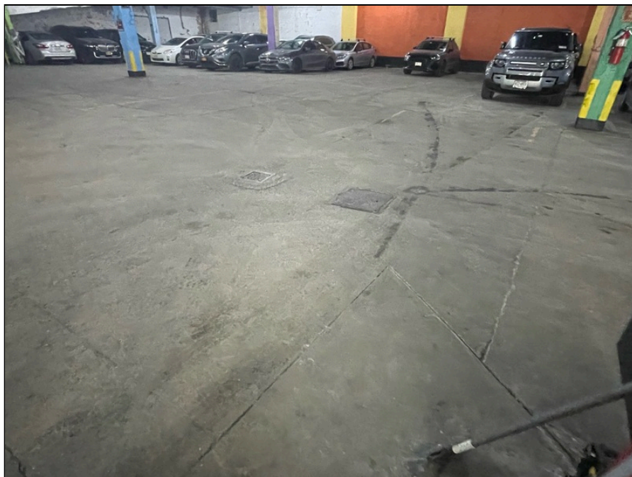
Photo 18: First floor parking garage finishes
