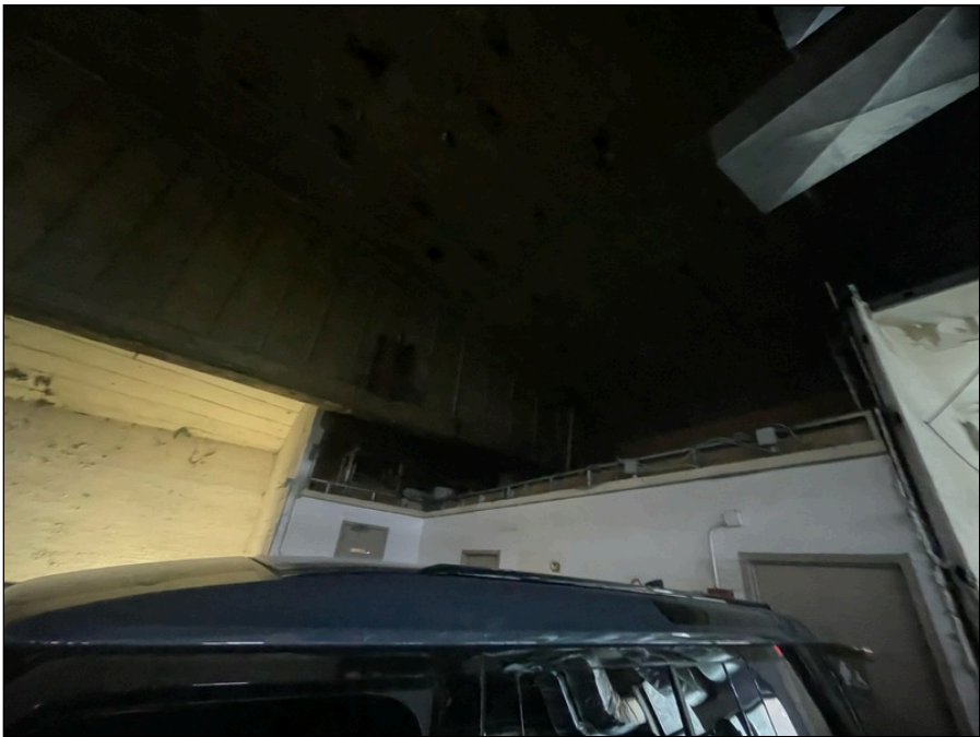
Photo 92: Second floor finishes
