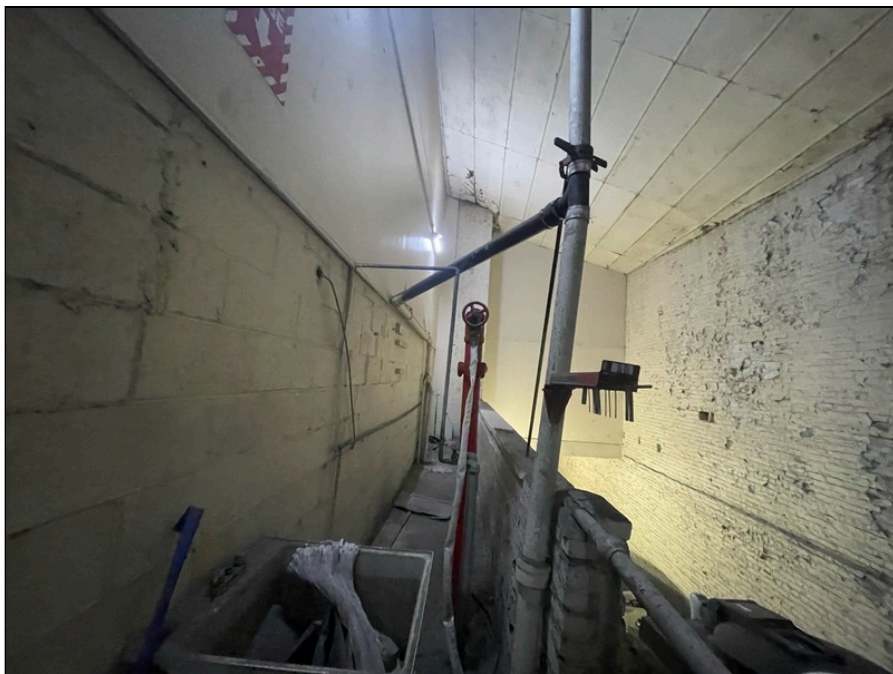
Photo 134: Second floor finishes
