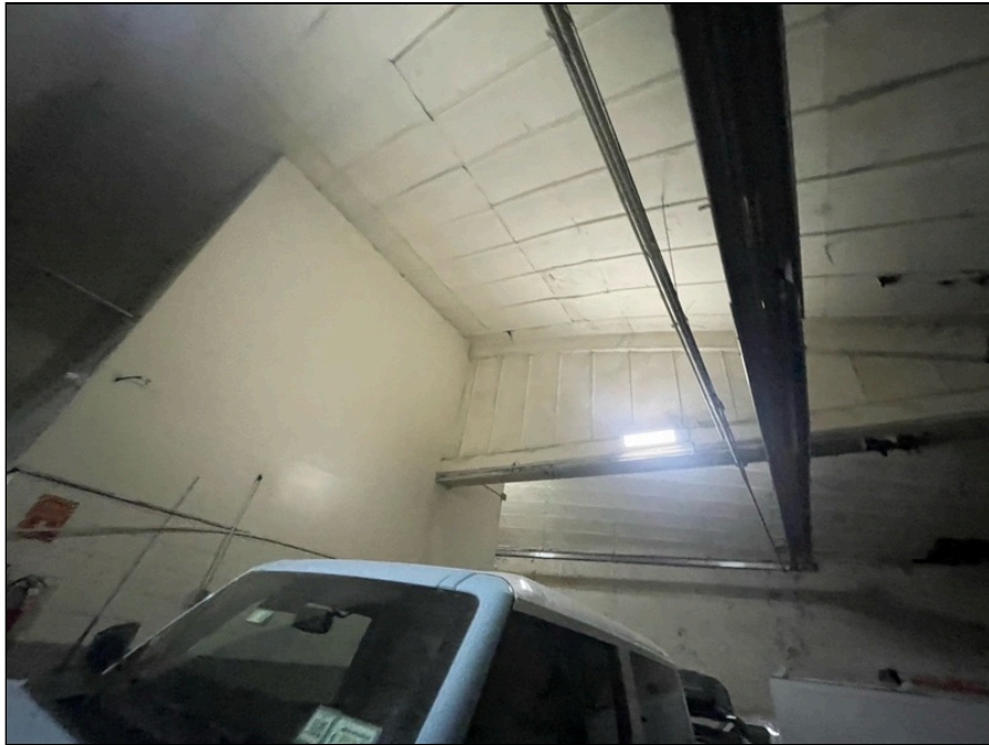
Photo 121: Second floor finishes
