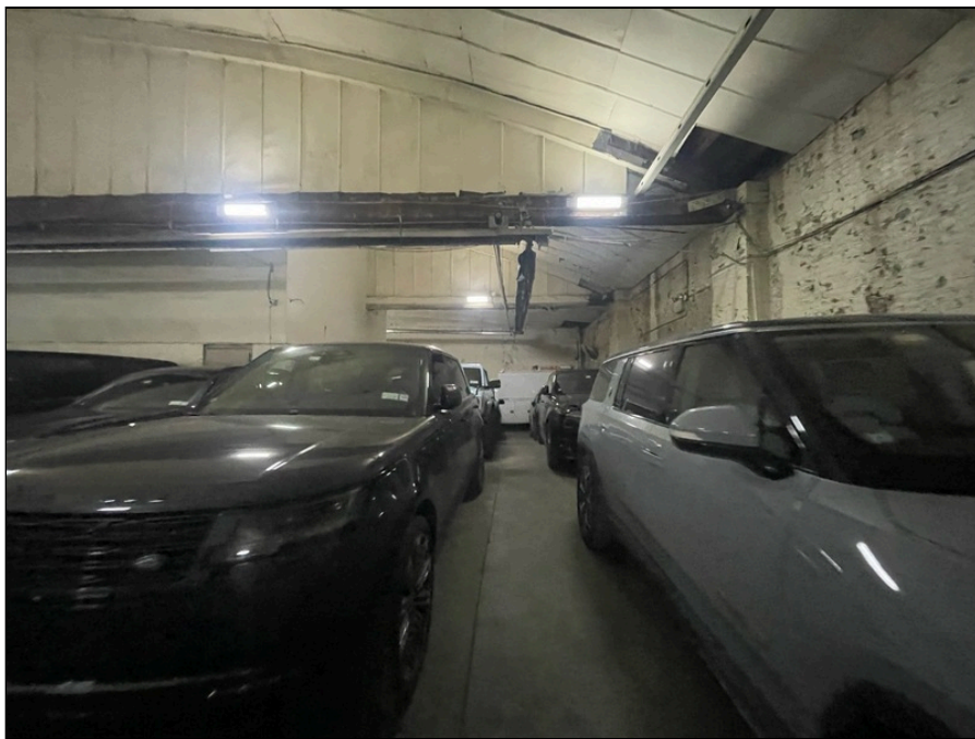
Photo 118: Second floor finishes
