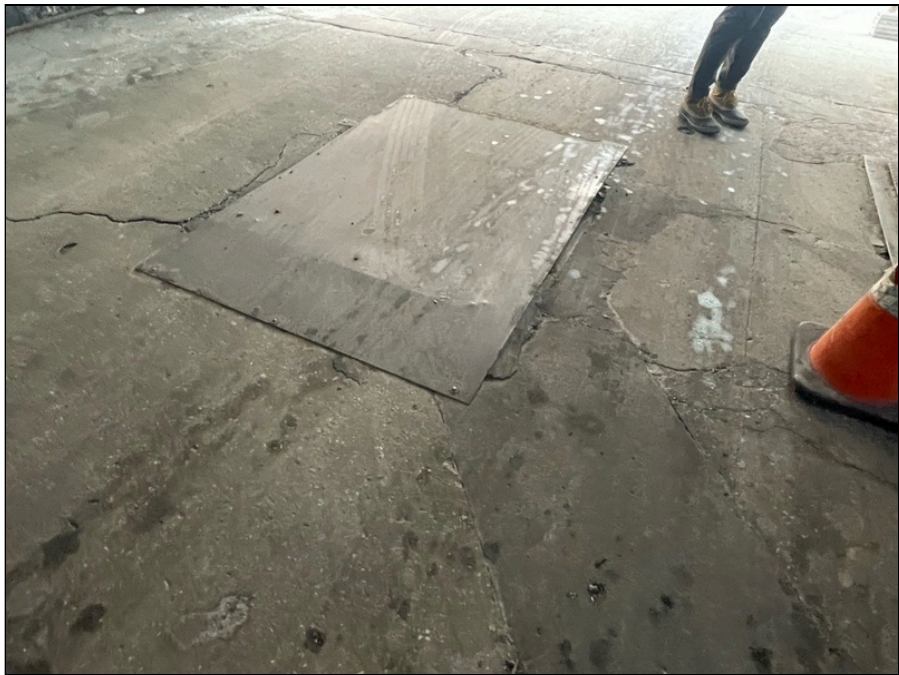
Photo 26: Oil-water separator, first floor
