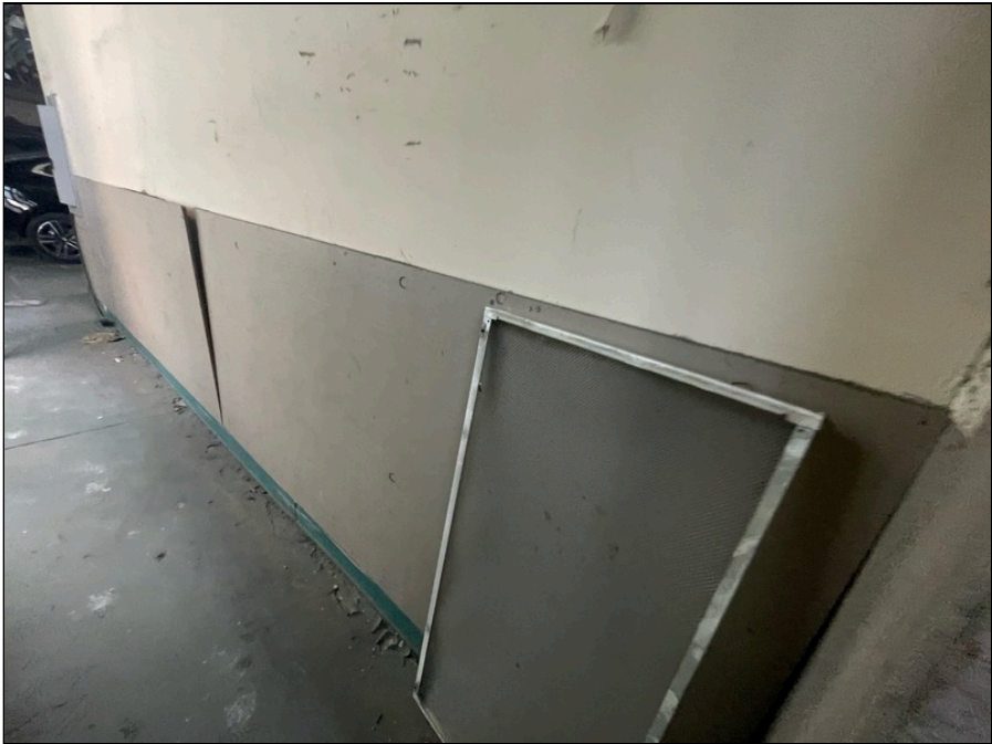
Photo 79: Second floor finishes
