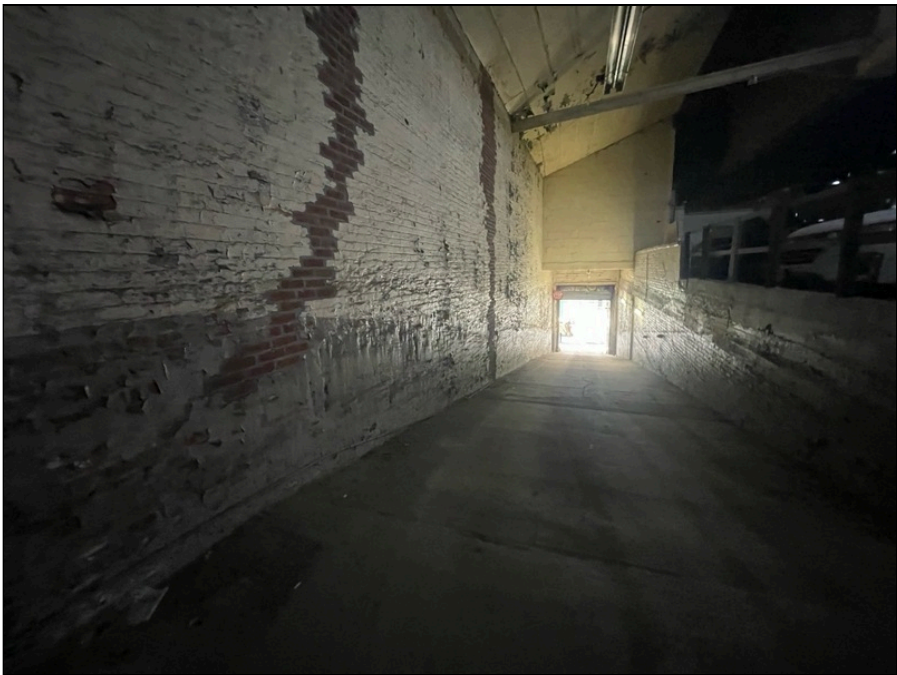
Photo 106: Second floor finishes
