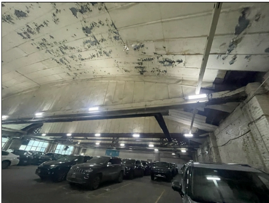
Photo 110: Second floor finishes
