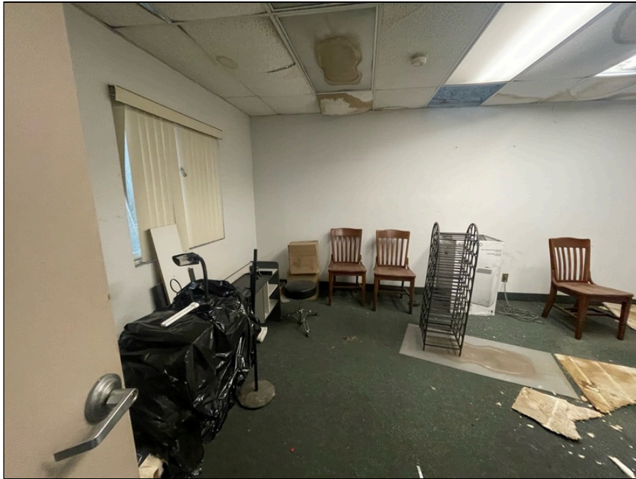
Photo 151: Second floor finishes
