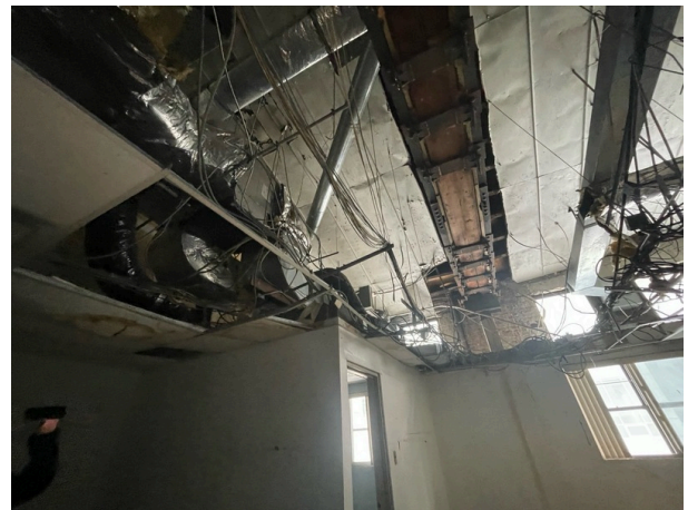
Second floor finishes
