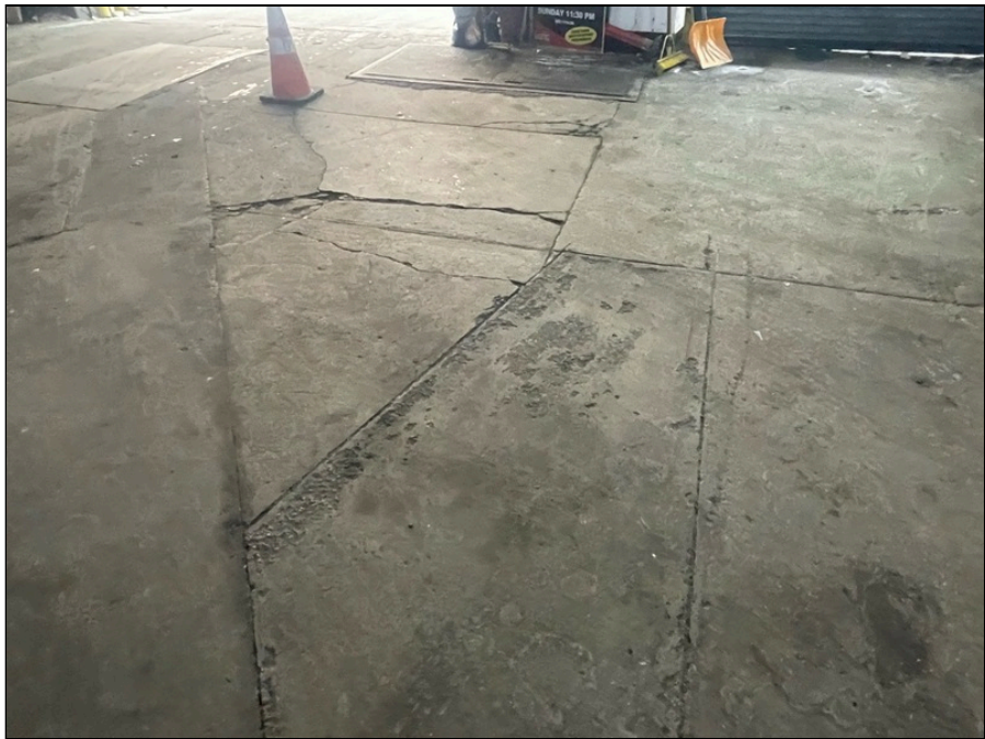
Photo 24: First floor parking garage finishes
