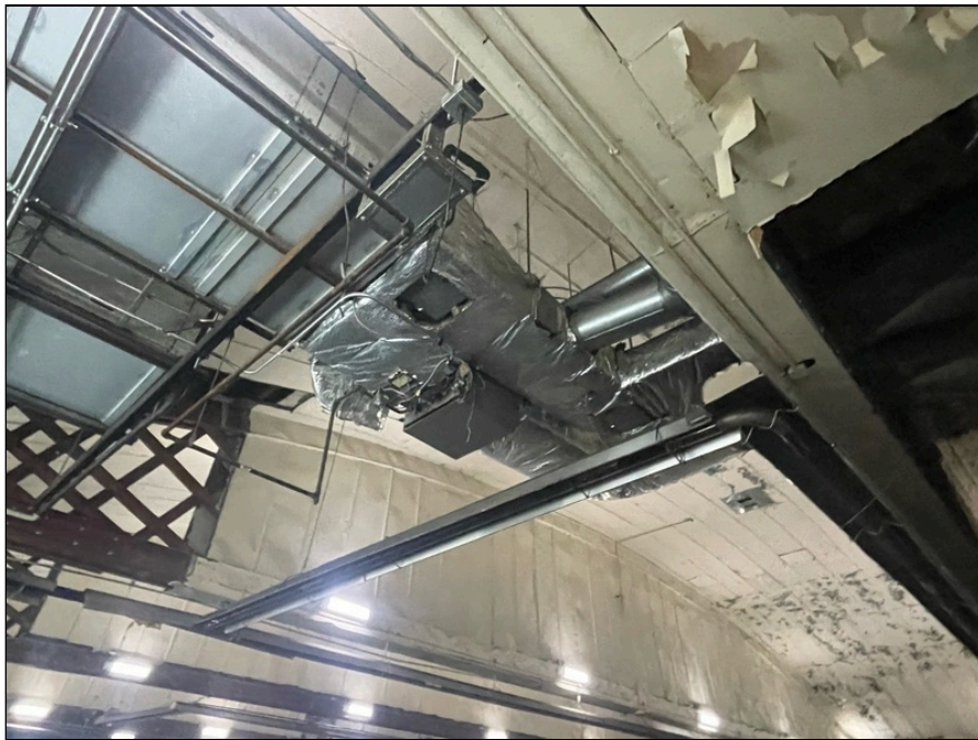
Photo 86: Second floor finishes
