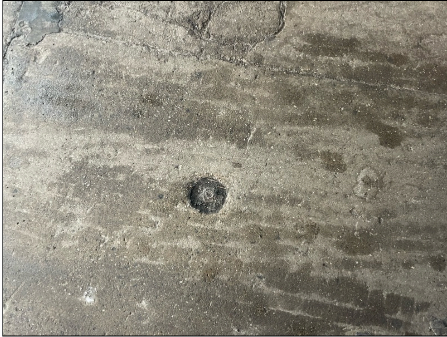
Photo 27: Floor drain cleanout, first floor
