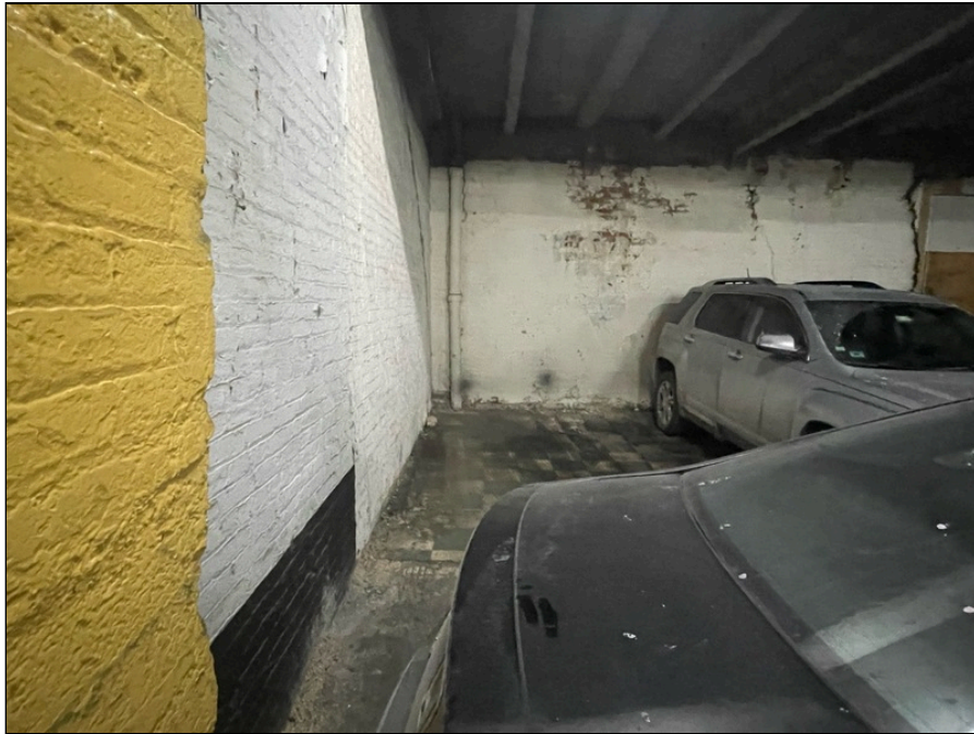
Photo 51: First floor parking garage finishes
