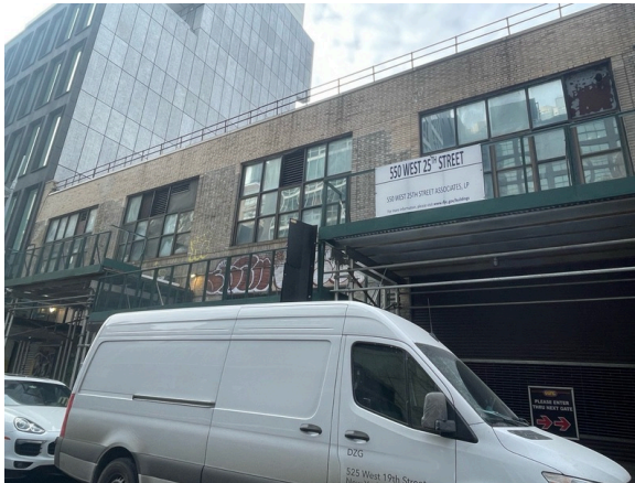
North side of the building
