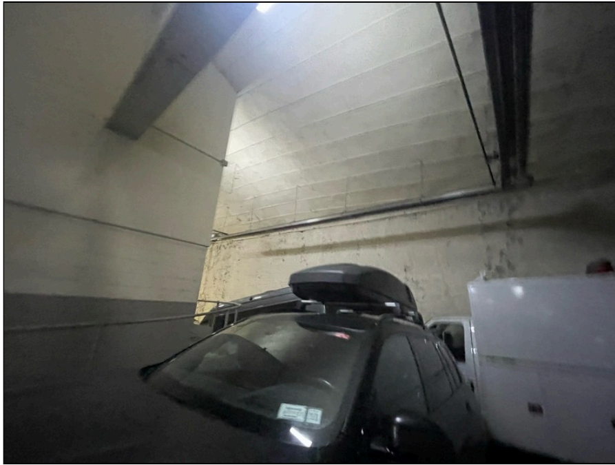
Photo 123: Second floor finishes
