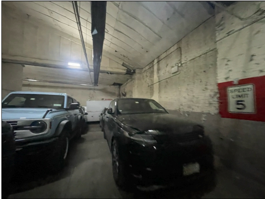
Photo 119: Second floor finishes
