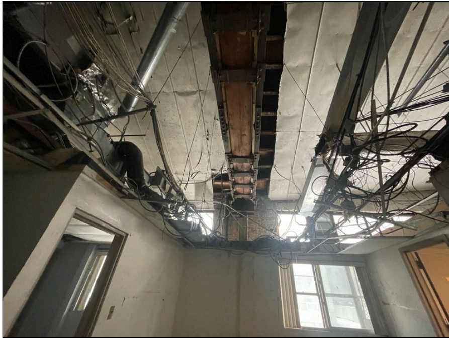
Photo 149: Second floor finishes
