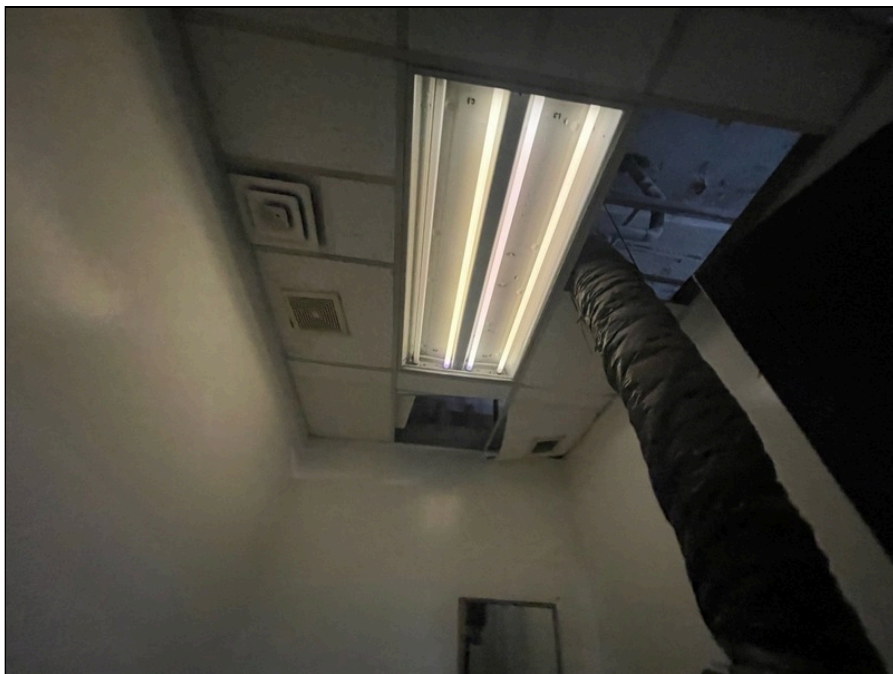
Photo 60: Bathroom finishes, first floor
