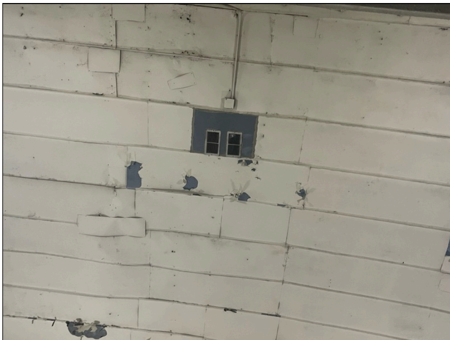
Photo 202: Second floor finishes
