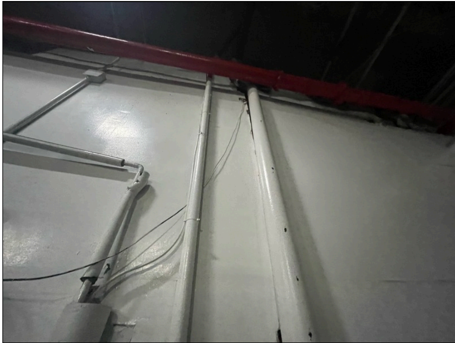
Photo 37: Roof drain piping, first floor
