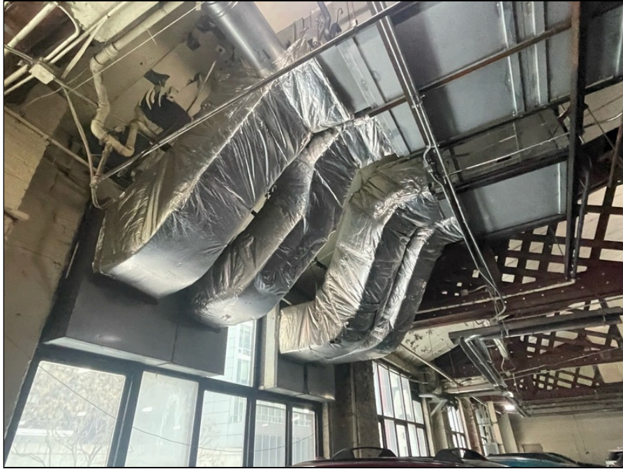
Photo 87: Second floor finishes
