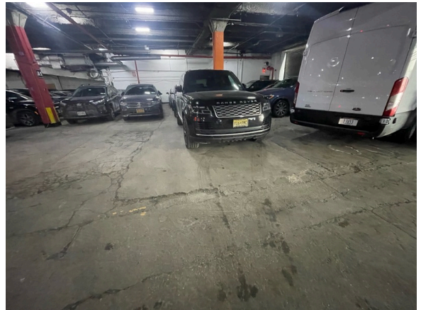
First floor parking garage finishes
