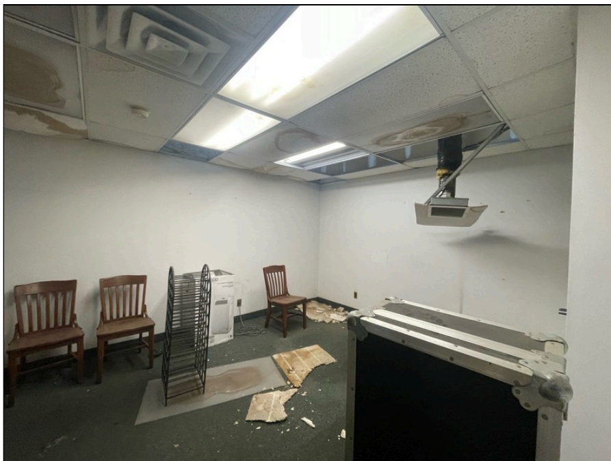
Photo 150: Second floor finishes
