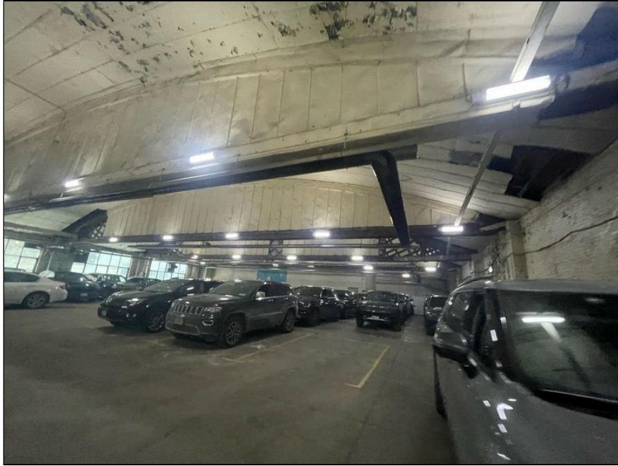
Photo 111: Second floor finishes
