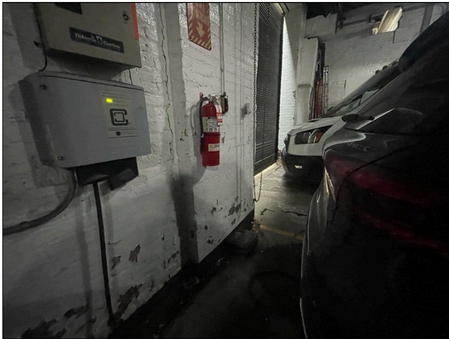
Photo 44: First floor parking garage finishes
