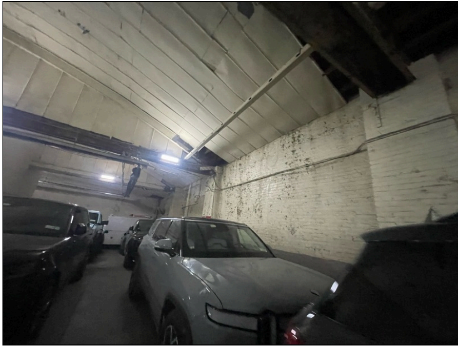
Photo 117: Second floor finishes
