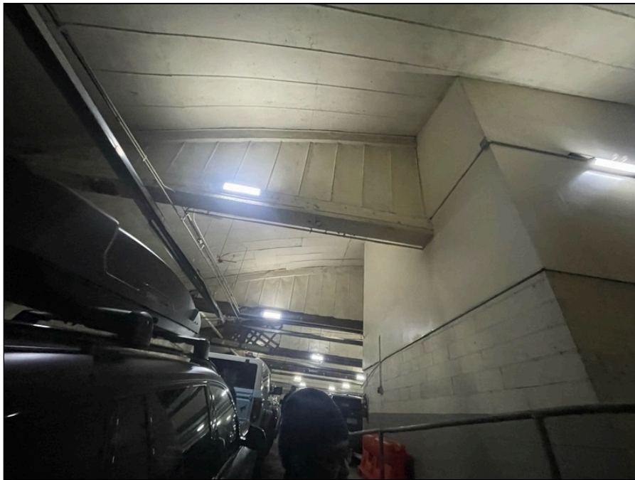
Photo 128: Second floor finishes
