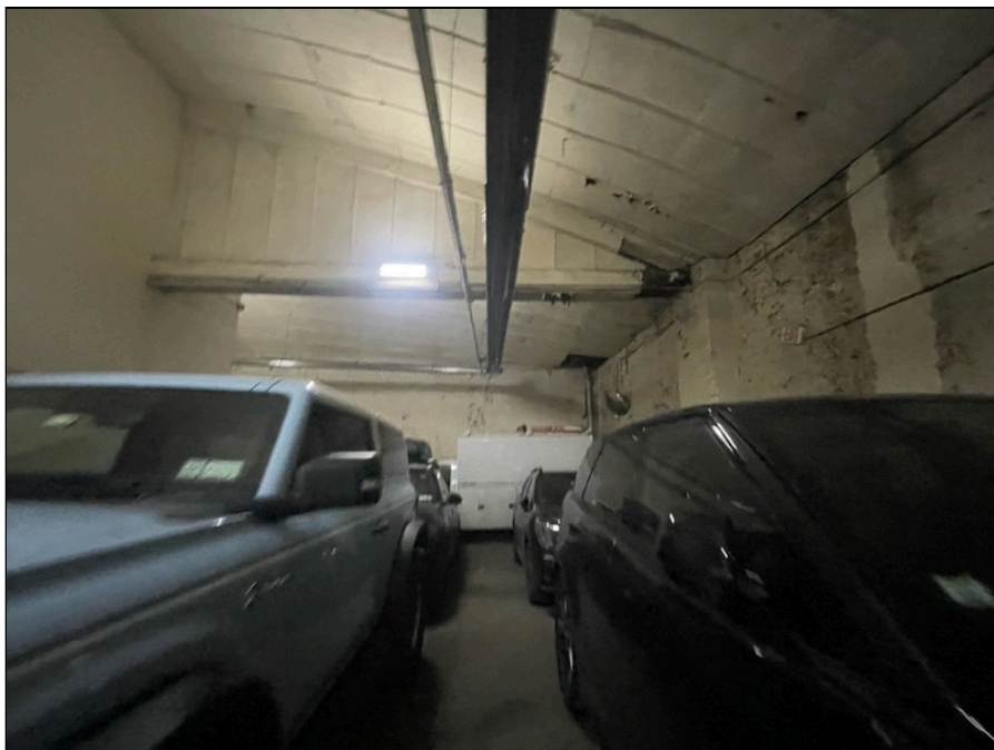
Photo 120: Second floor finishes
