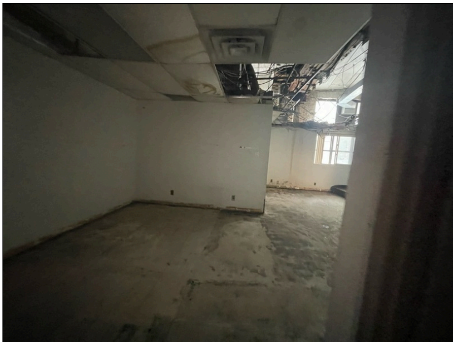
Photo 144: Second floor finishes
