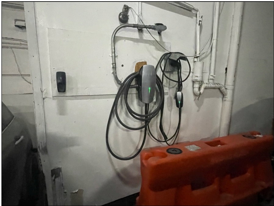
Photo 34: First floor parking garage finishes
