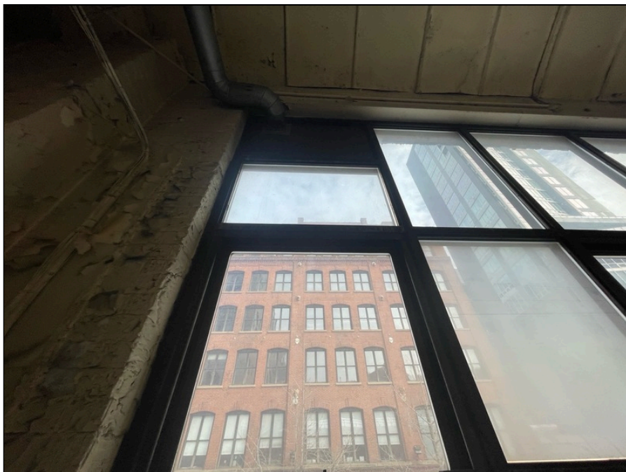
Photo 82: Second floor finishes
