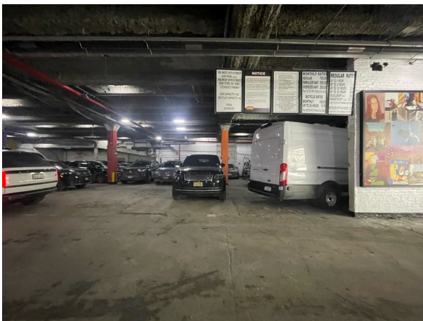
First floor parking garage finishes
