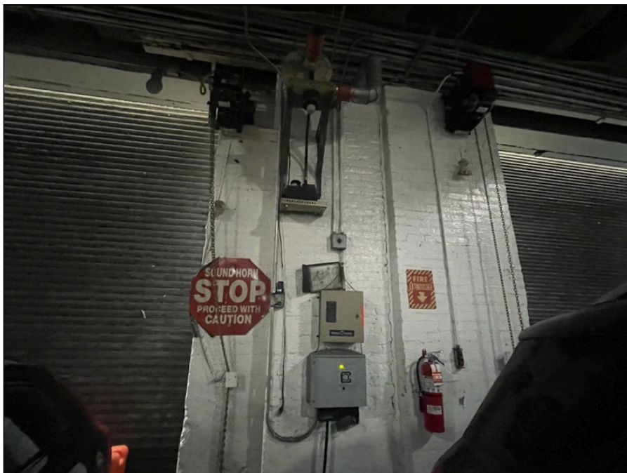
Photo 42: First floor parking garage finishes
