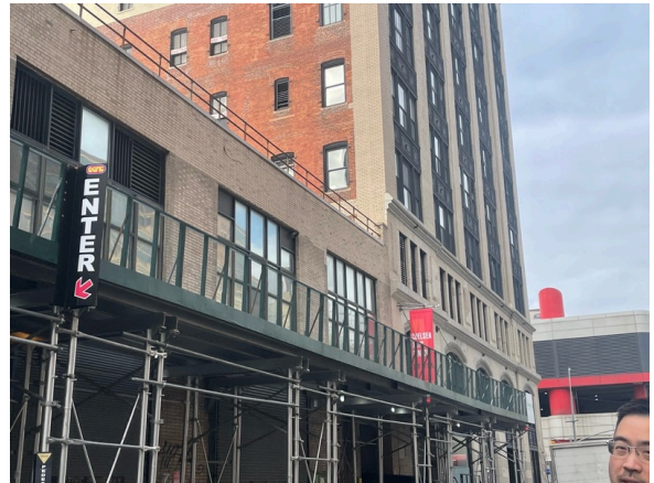
North side of the building
