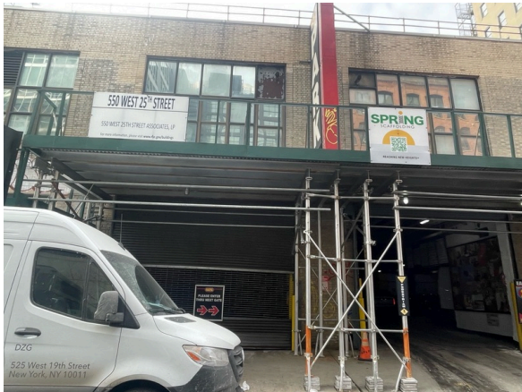
North side of the building
