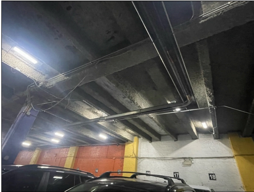
Photo 47: Floor drain, first floor
