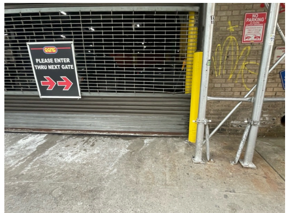
North side of the building
