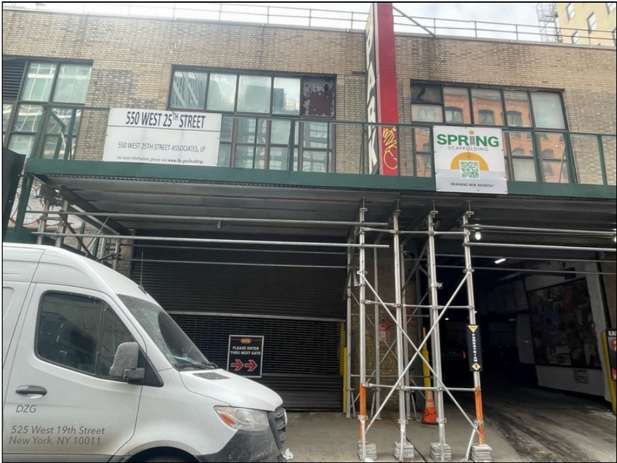
Photo 2: North side of the building
