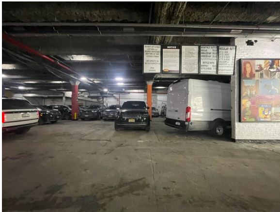
First floor parking garage finishes
