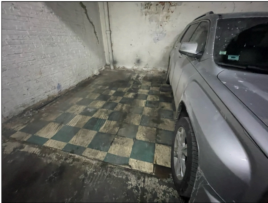
Photo 54: First floor parking garage finishes
