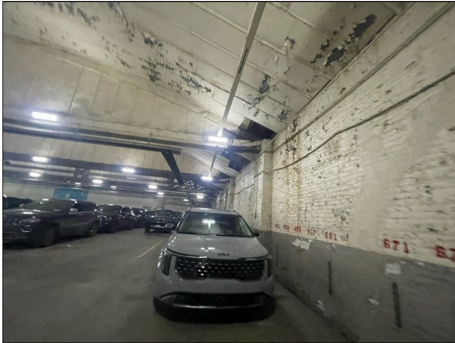
Photo 109: Second floor finishes
