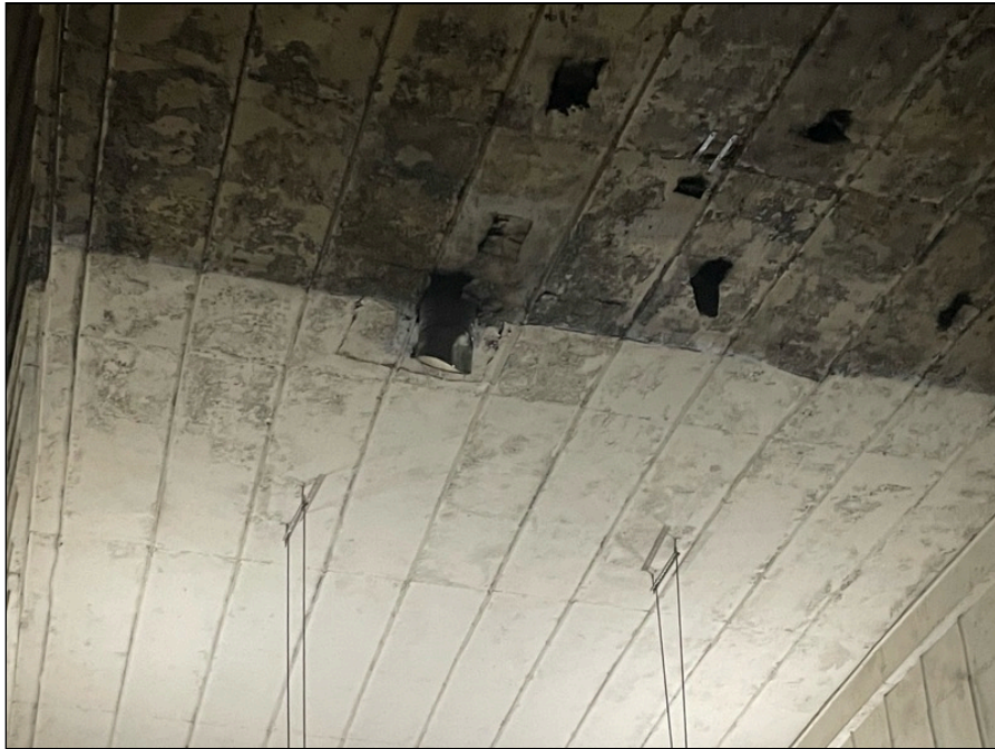
Photo 201: Second floor finishes
