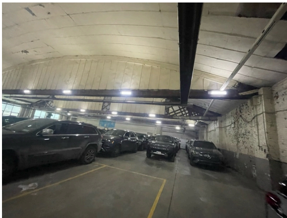
Second floor finishes
