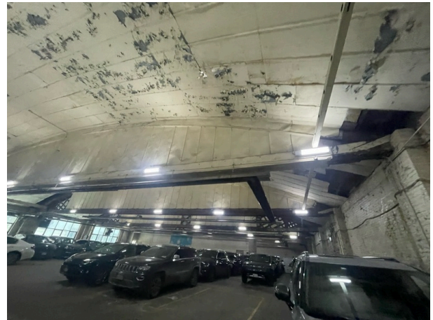
Second floor finishes
