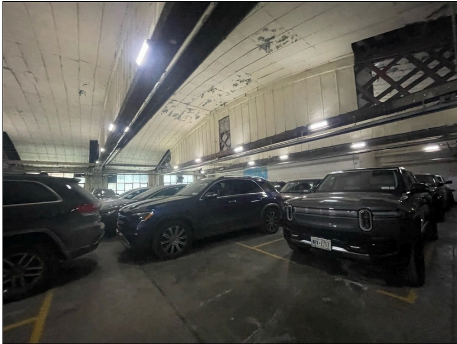
Photo 115: Second floor finishes
