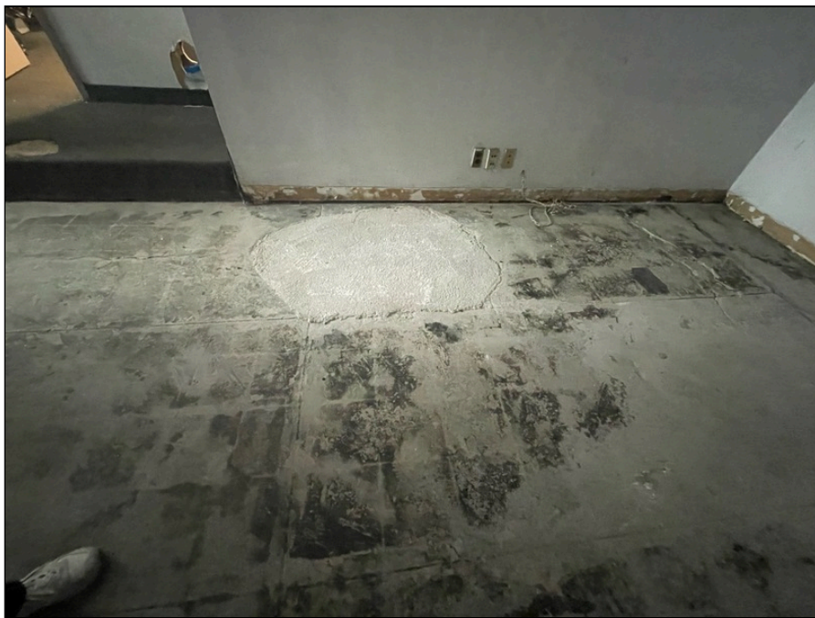
Photo 156: Second floor finishes
