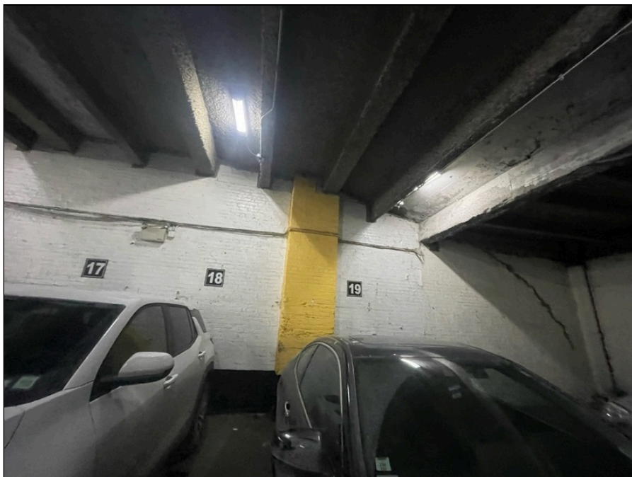
Photo 50: First floor parking garage finishes
