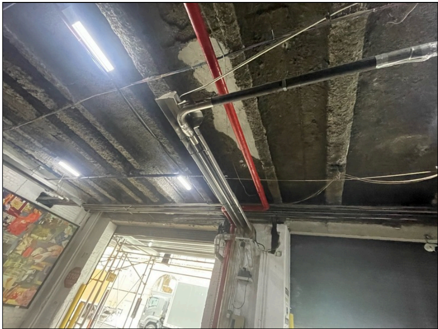
Photo 12: First floor parking garage finishes
