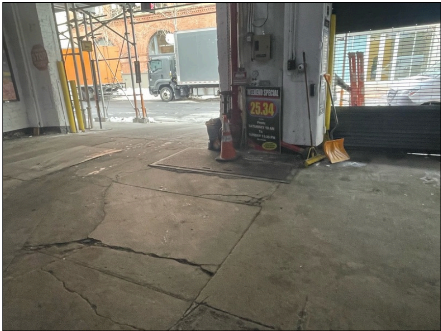
Photo 14: Sewer and water connections, first floor
