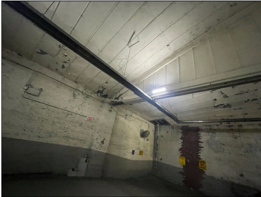
Photo 103: Second floor finishes
