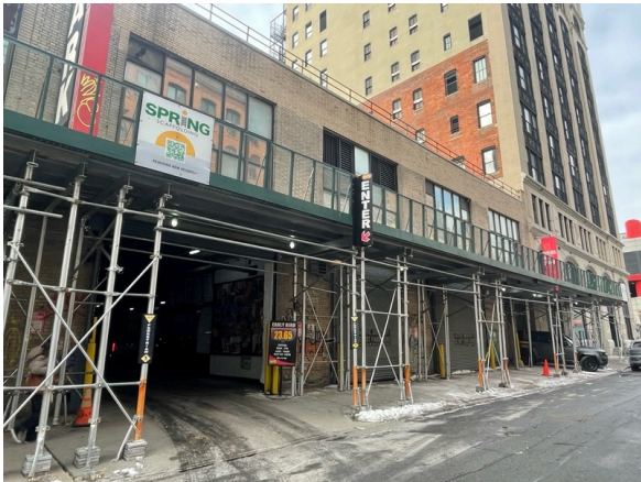
North side of the building
