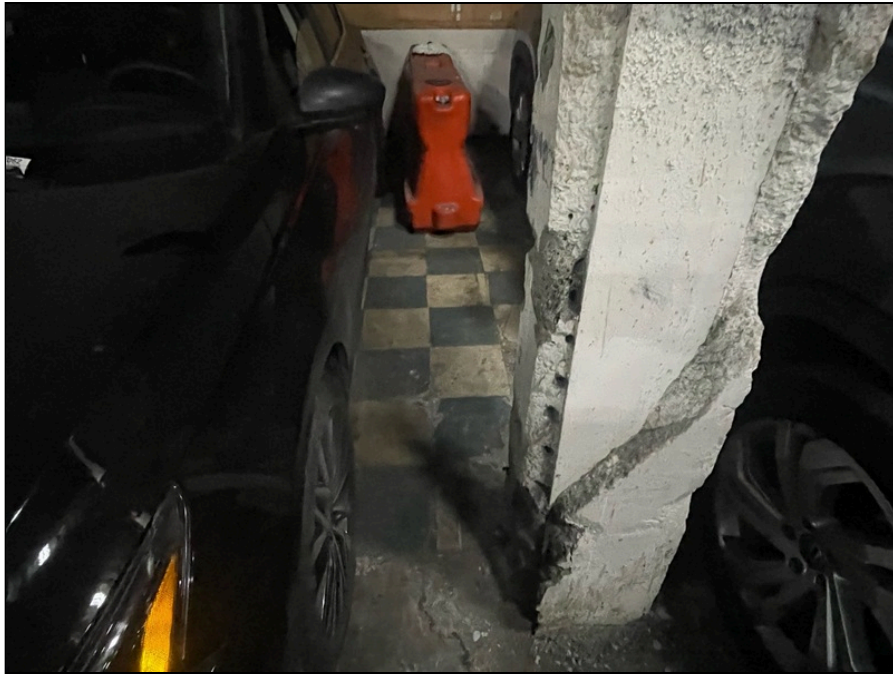
Photo 53: First floor parking garage finishes
