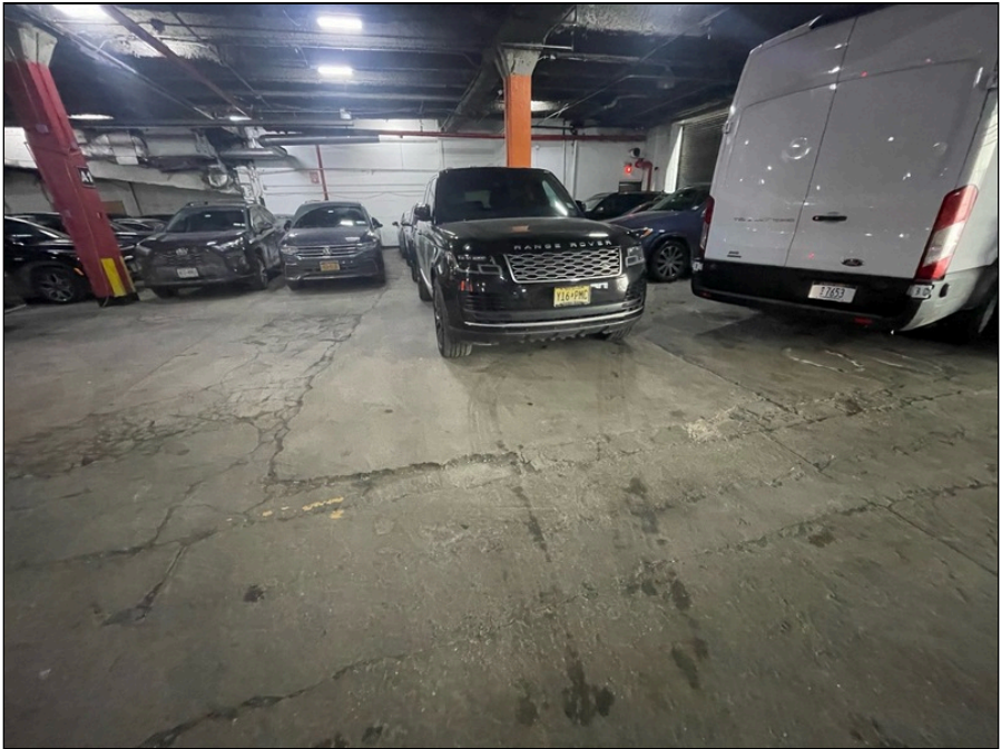
Photo 31: First floor parking garage finishes
