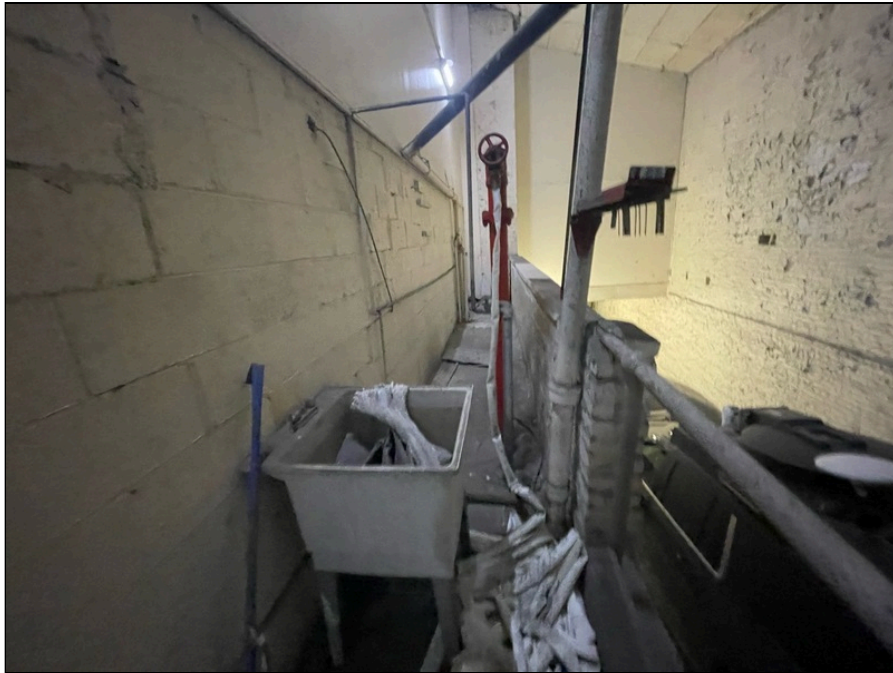
Photo 131: Second floor finishes
