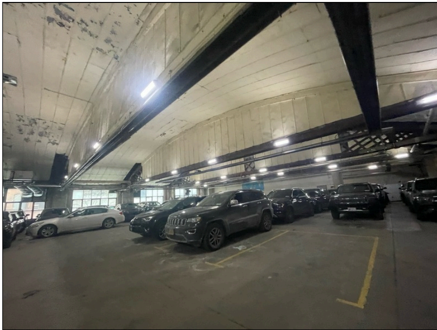
Photo 112: Second floor finishes
