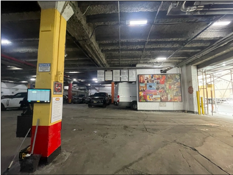
Photo 9: First floor parking garage finishes
