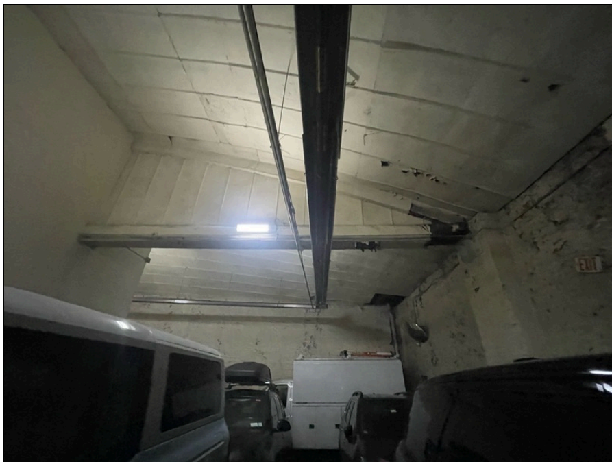
Photo 122: Second floor finishes
