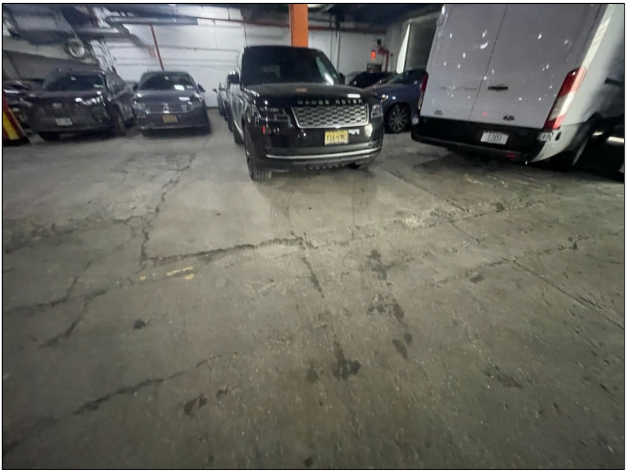
Photo 32: First floor parking garage finishes
