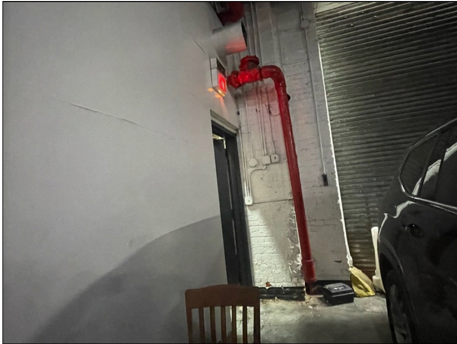
Photo 41: First floor parking garage finishes
