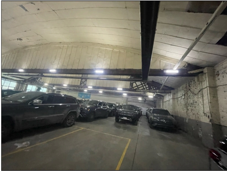
Photo 113: Second floor finishes
