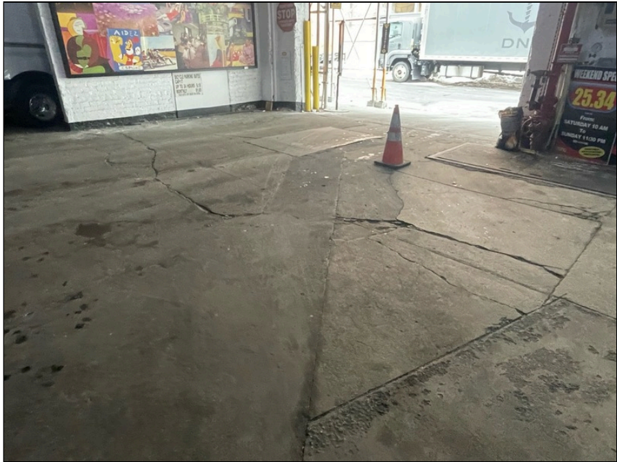
Photo 25: First floor parking garage finishes
