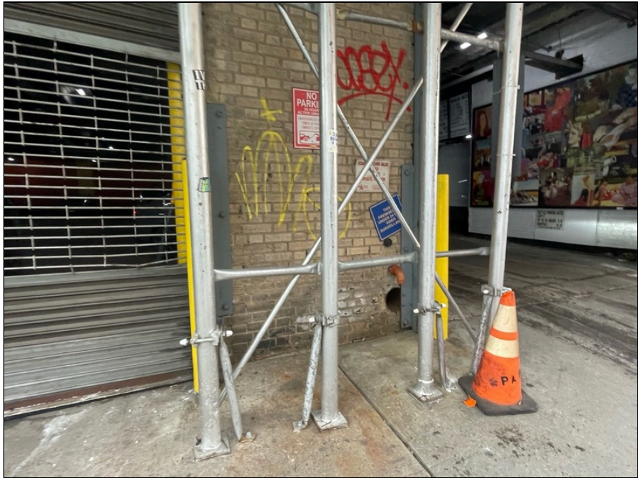
Photo 7: North side of the building
