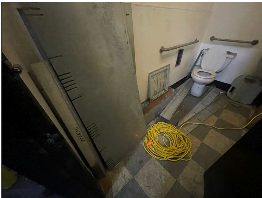
Photo 57: Bathroom finishes, first floor
