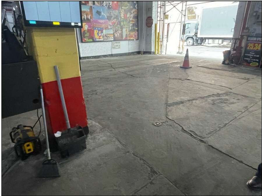
Photo 23: First floor parking garage finishes
