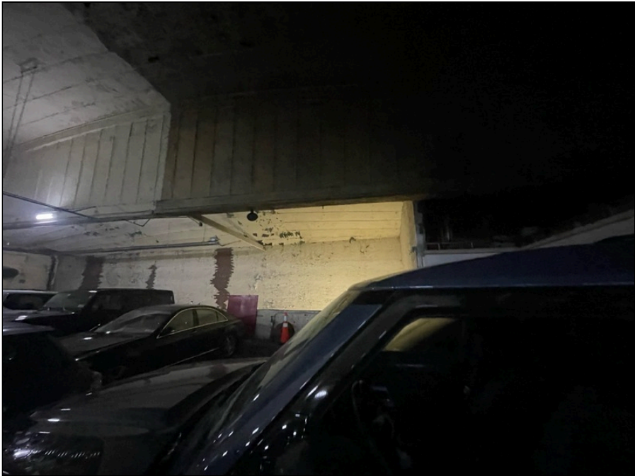
Photo 93: Second floor finishes
