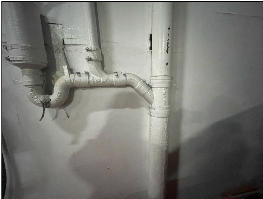
Photo 36: Roof drain piping, first floor
