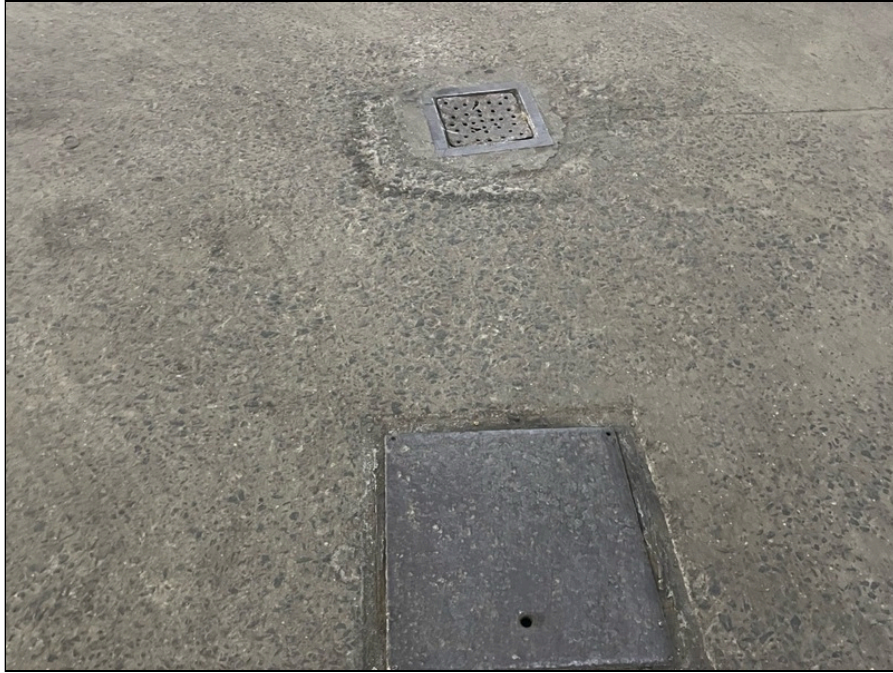
Photo 19: Floor drain, first floor
