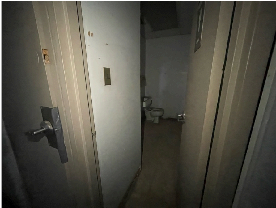
Photo 143: Second floor finishes
