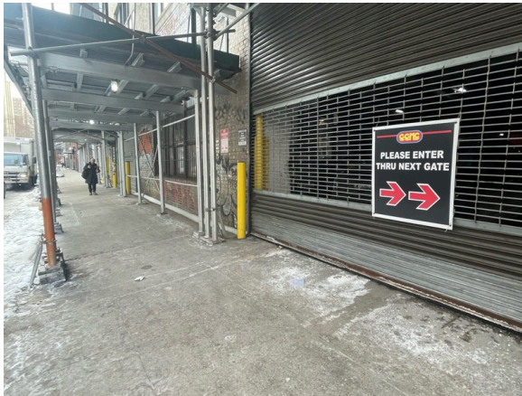
North side of the building
