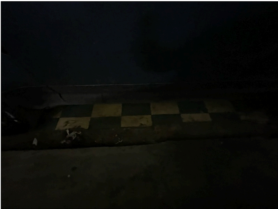
Photo 94: Second floor finishes
