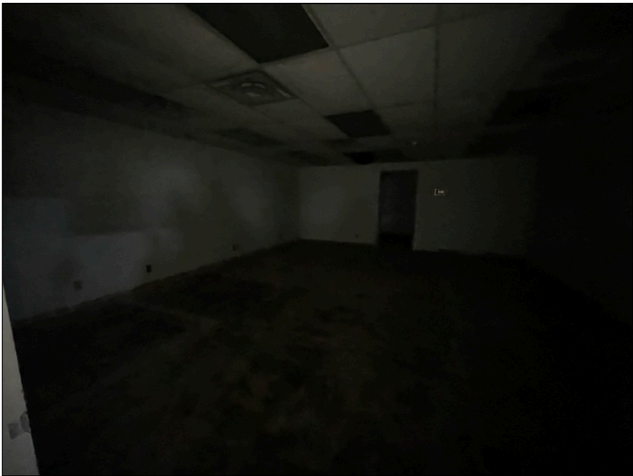
Photo 142: Second floor finishes
