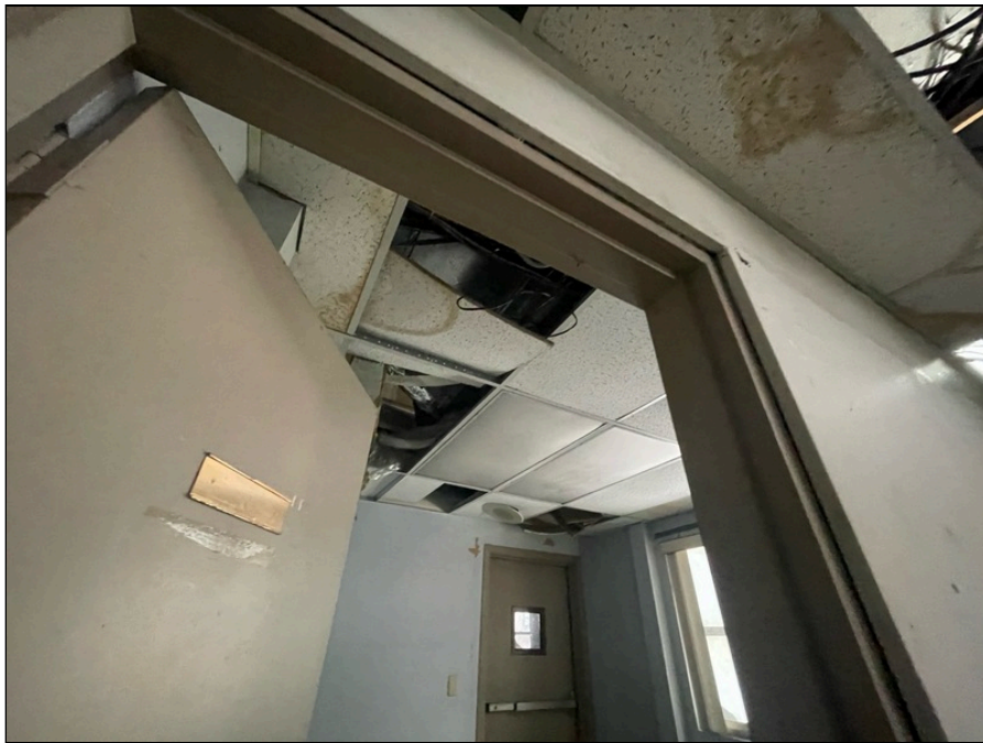
Photo 154: Second floor finishes
