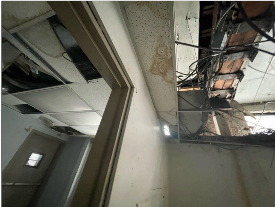
Photo 155: Second floor finishes
