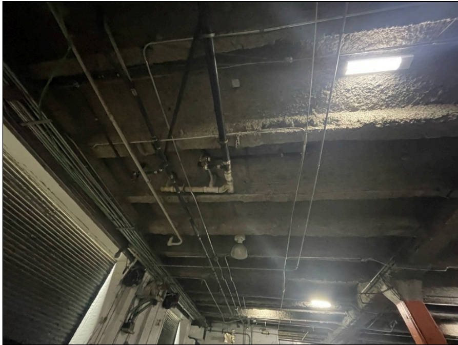
Photo 39: First floor parking garage finishes
