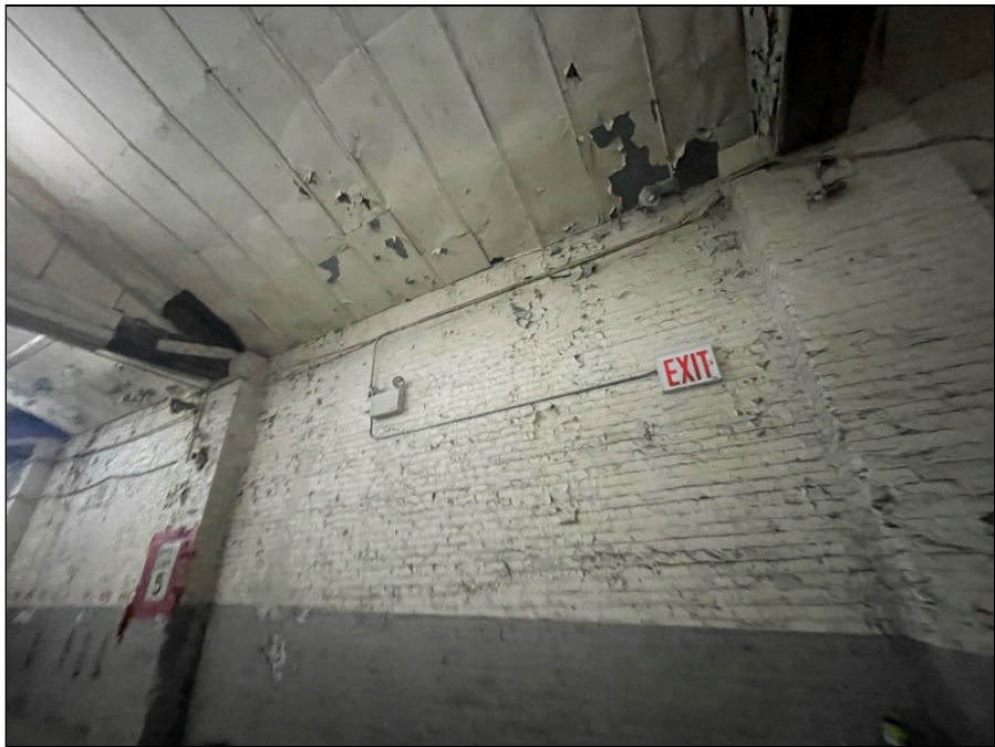
Photo 108: Second floor finishes
