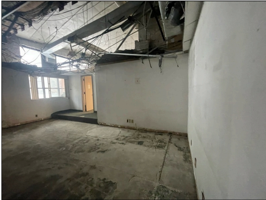
Photo 145: Second floor finishes
