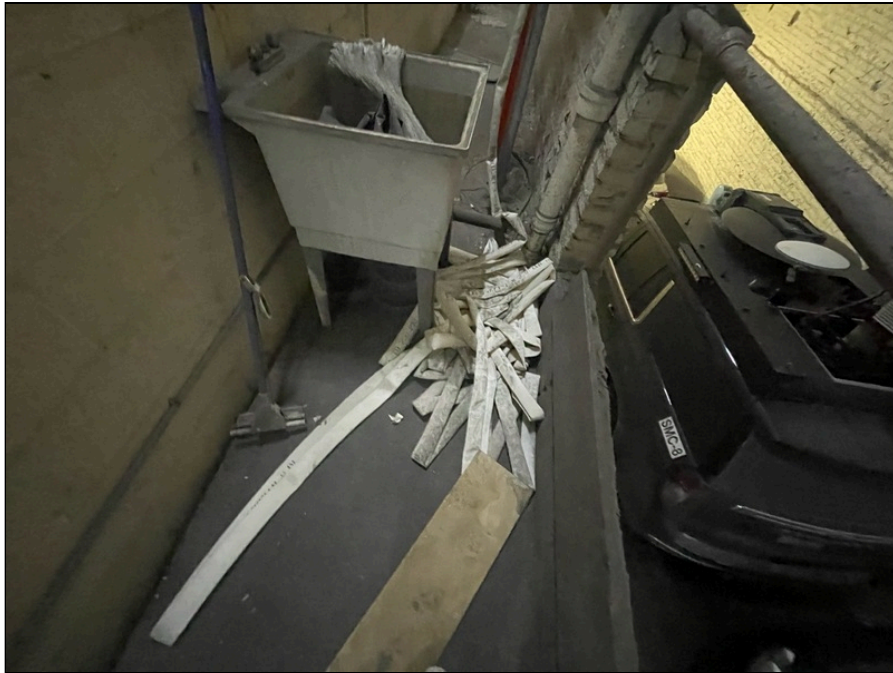
Photo 133: Second floor finishes
