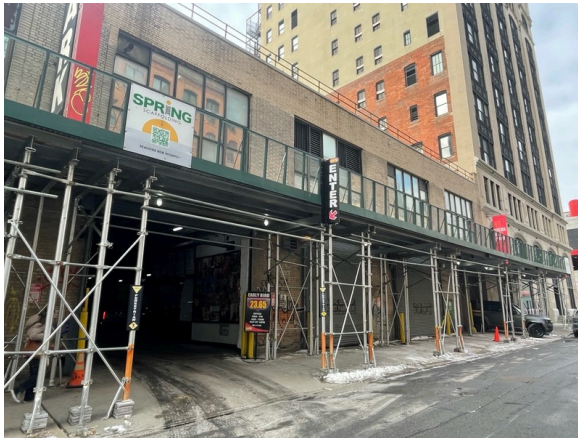
North side of the building
