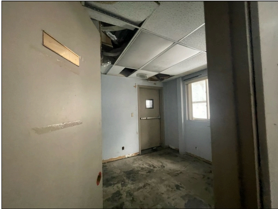
Photo 153: Second floor finishes
