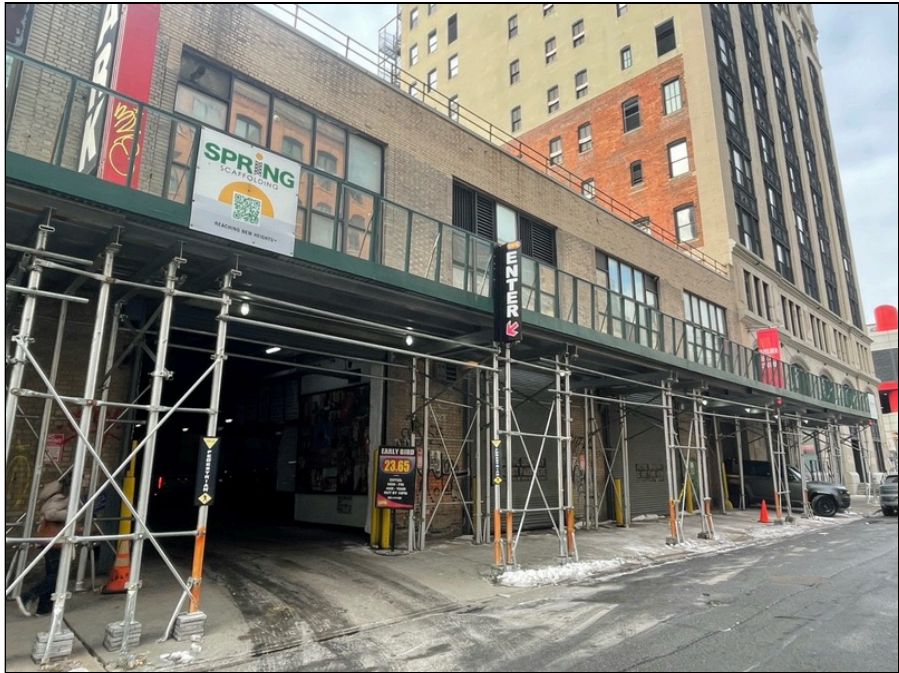
Photo 3: North side of the building
