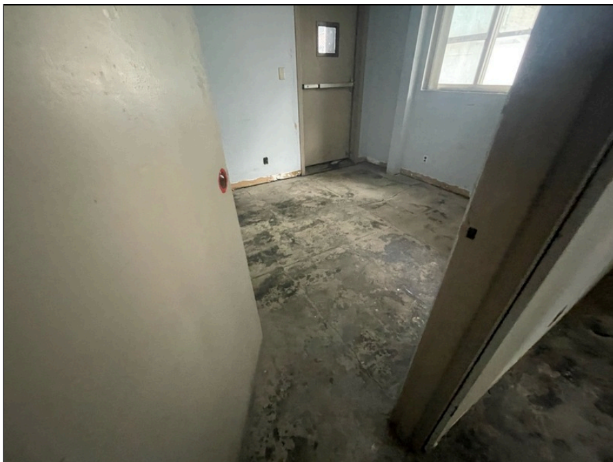
Photo 152: Second floor finishes
