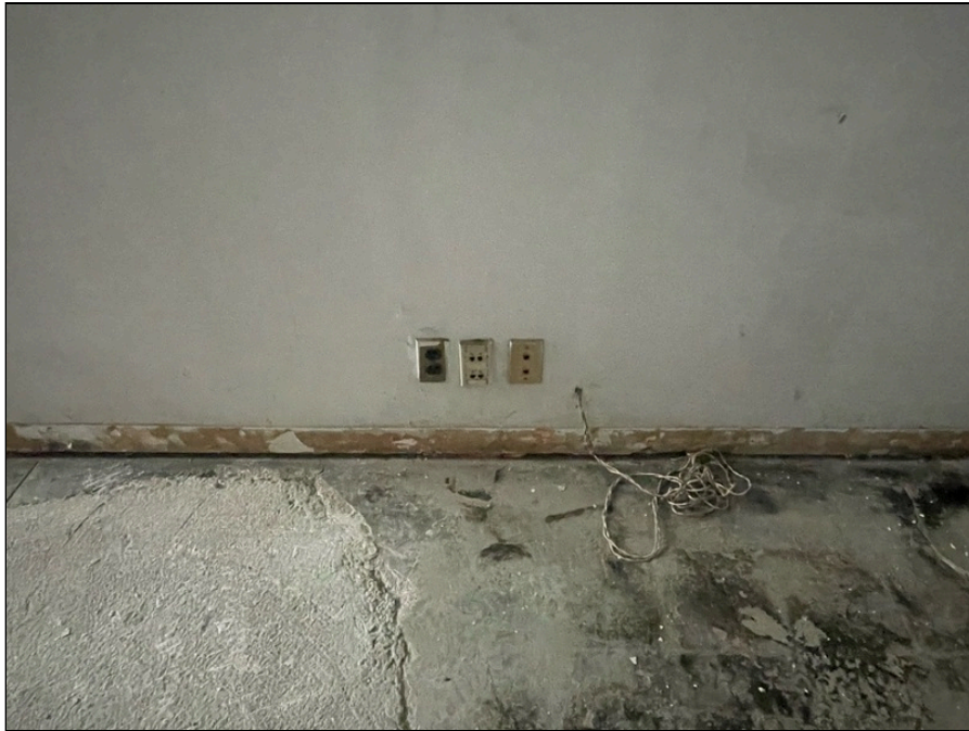
Photo 157: Second floor finishes
