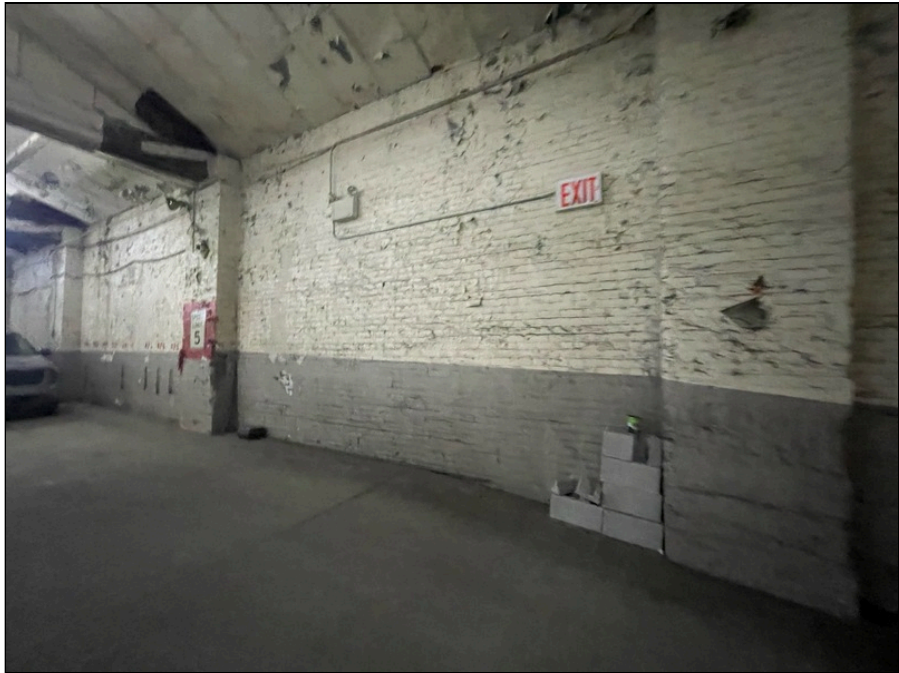
Photo 107: Second floor finishes
