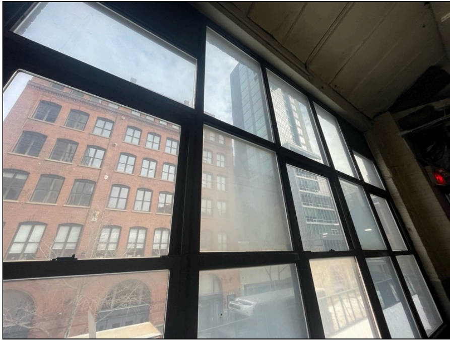
Photo 83: Second floor finishes
