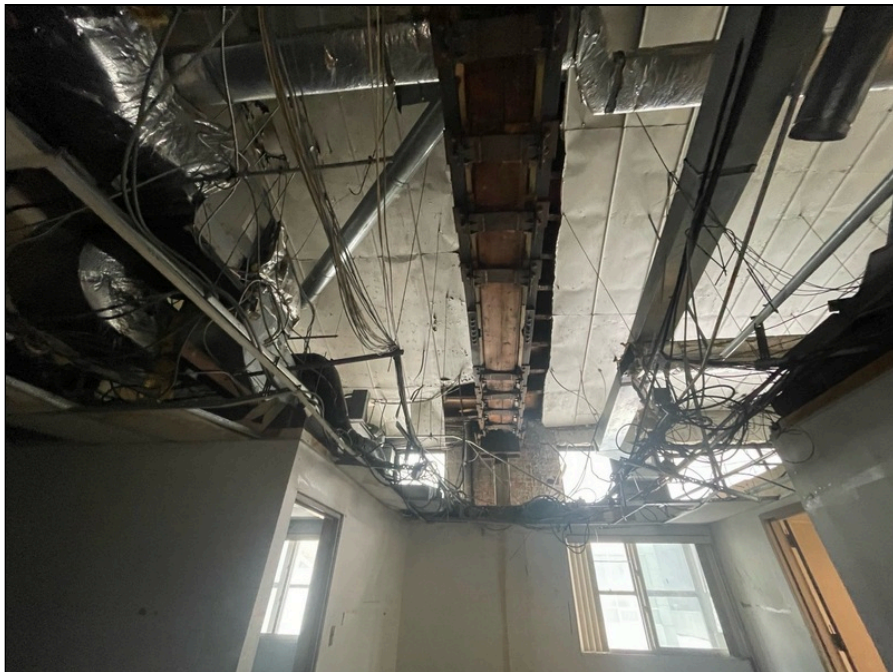
Photo 148: Second floor finishes
