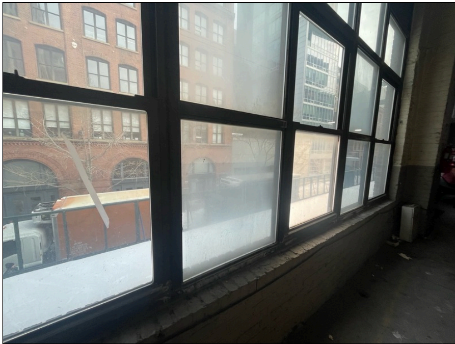
Photo 84: Second floor finishes
