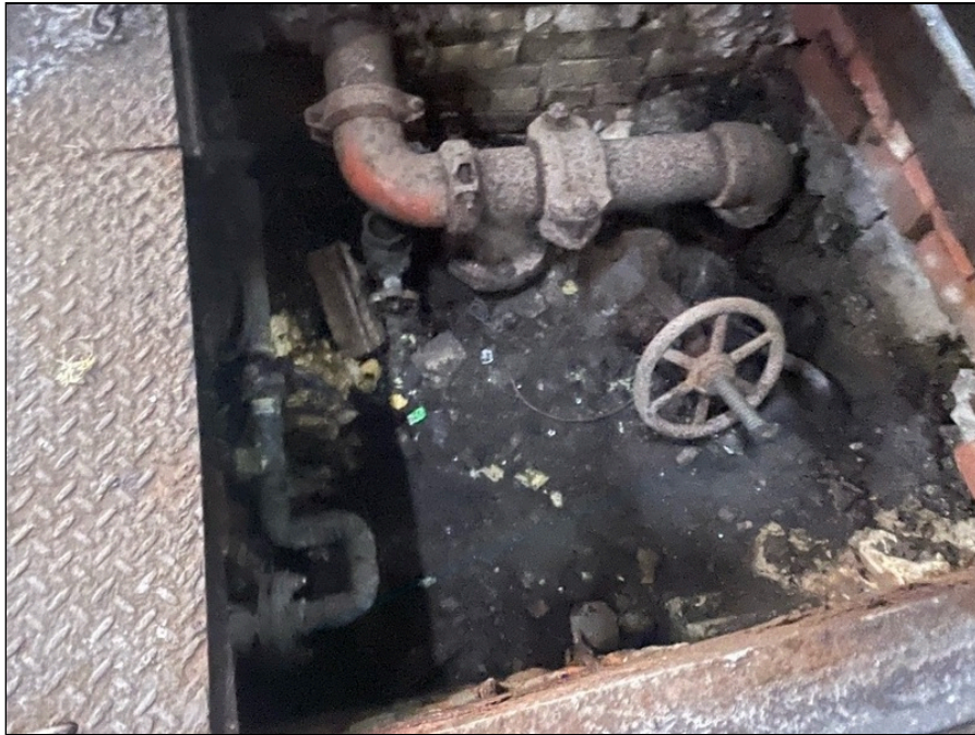
Photo 15: Sewer and water connections, first floor
