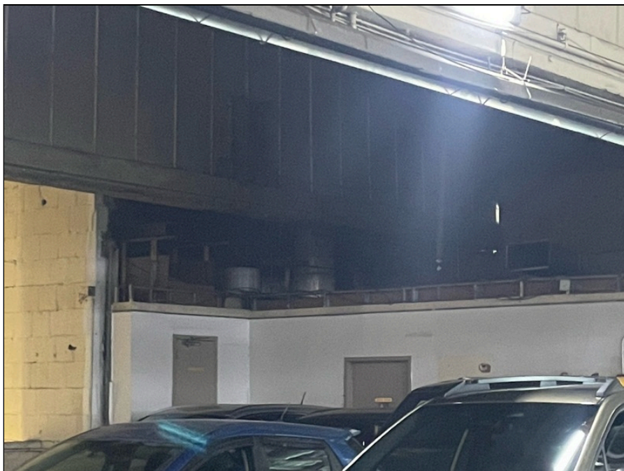
Photo 135: Hot water heaters, second floor
