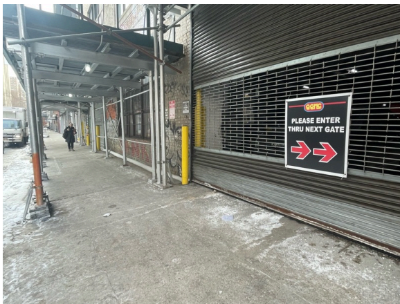
North side of the building
