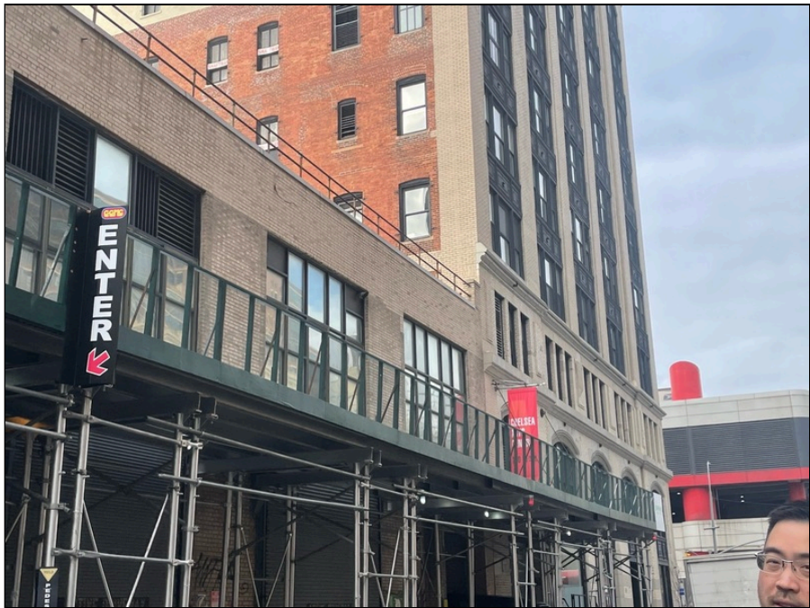
Photo 4: North side of the building
