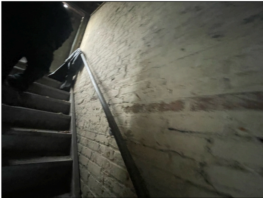
Photo 176: Stairwell to the roof
