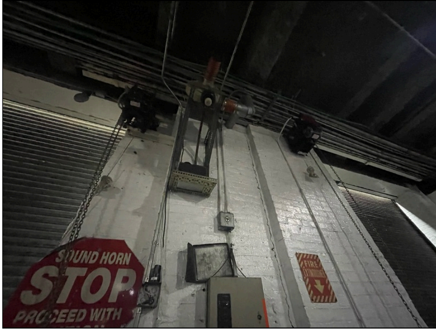
Photo 43: First floor parking garage finishes
