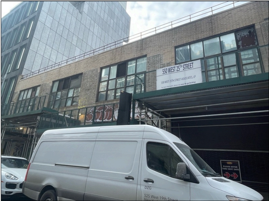
Photo 1: North side of the building
